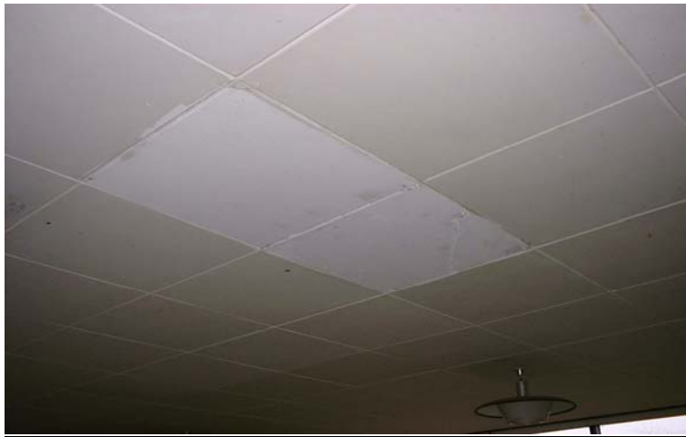
Fig 6: Asbestos Containing Ceiling Panels.
