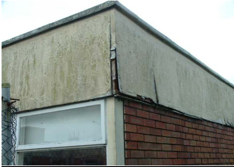
Fig 6: Asbestos Containing Ceiling Panels.
