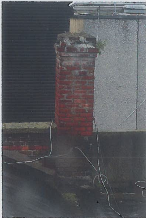
Photo 05 – View of chimney
