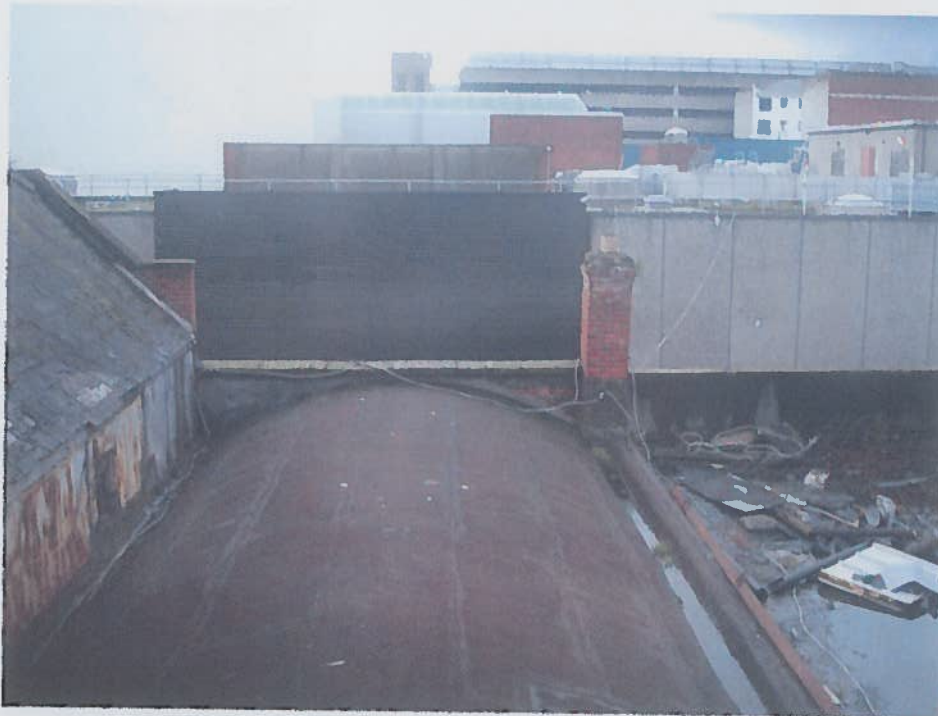
Photo 06 – External view of roof
