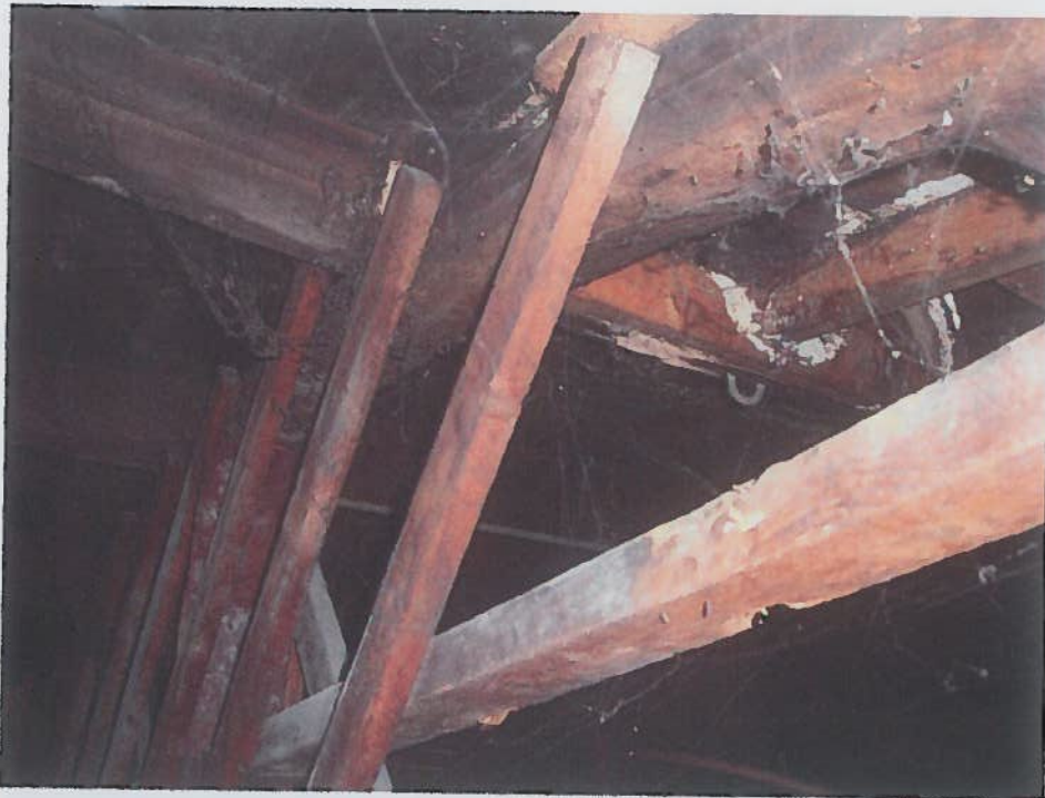
Photo 07 – Internal view of curved truss.
