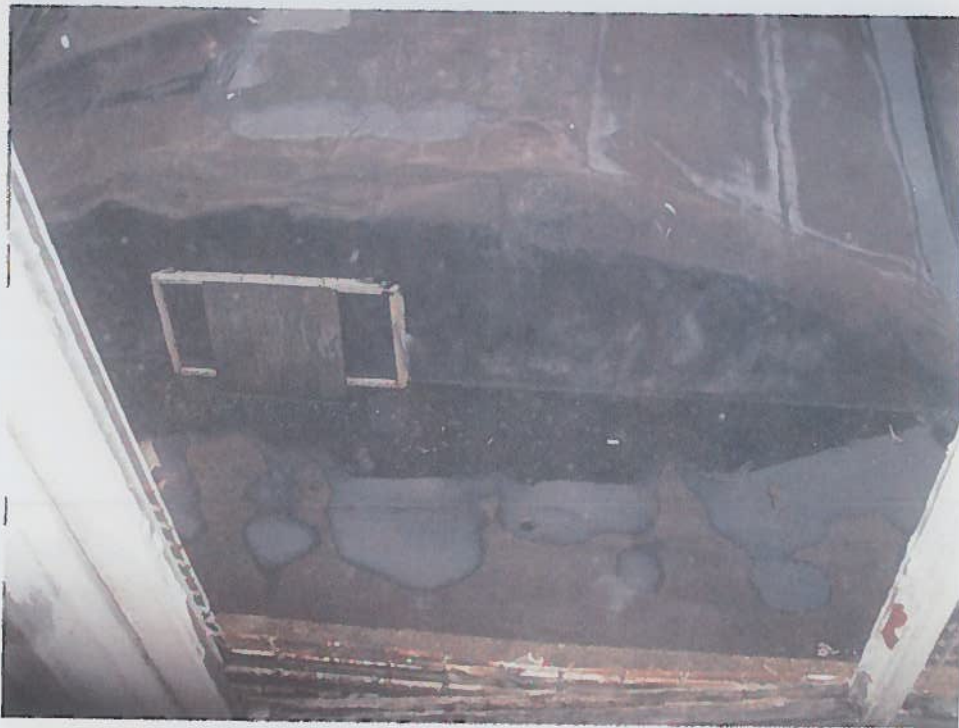
Photo 08 – External rear view of roof.
