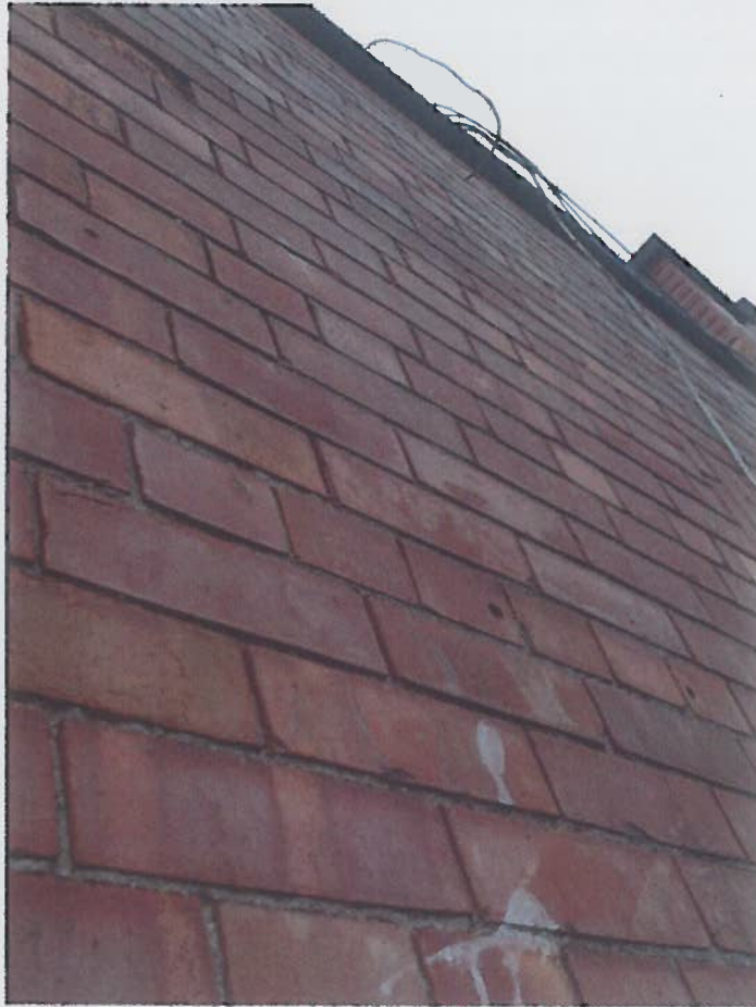
Photo. 03 – Brick detail to front elevation.
