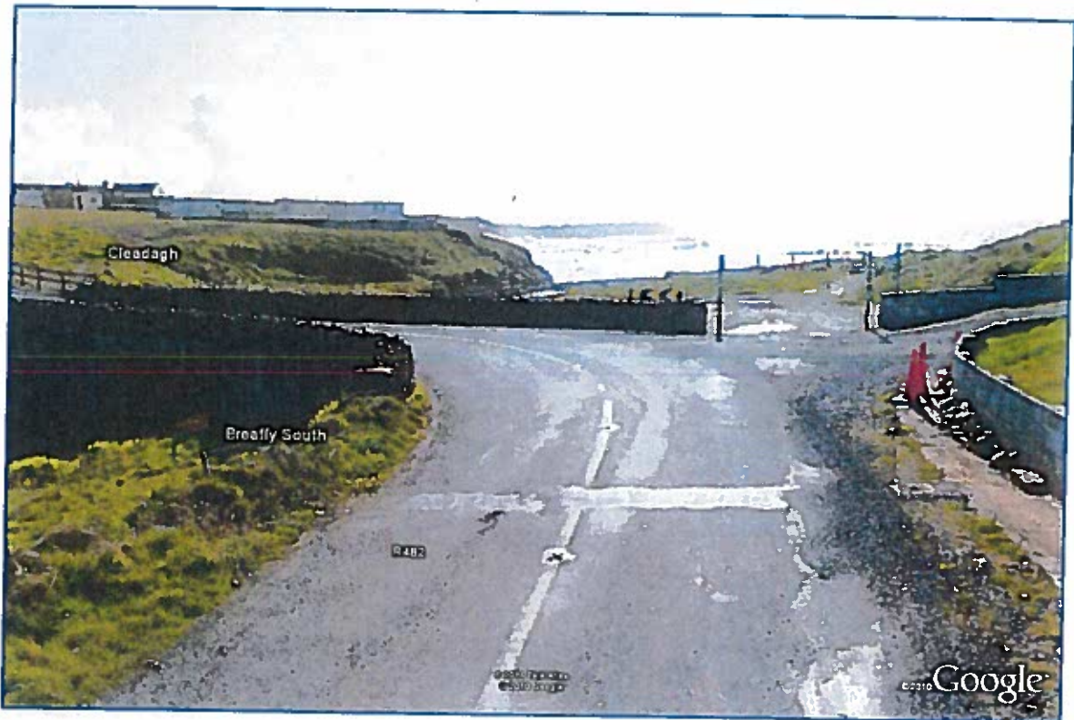
Plate 5.3 – Photo Location 3, Cleedagh Bridge
