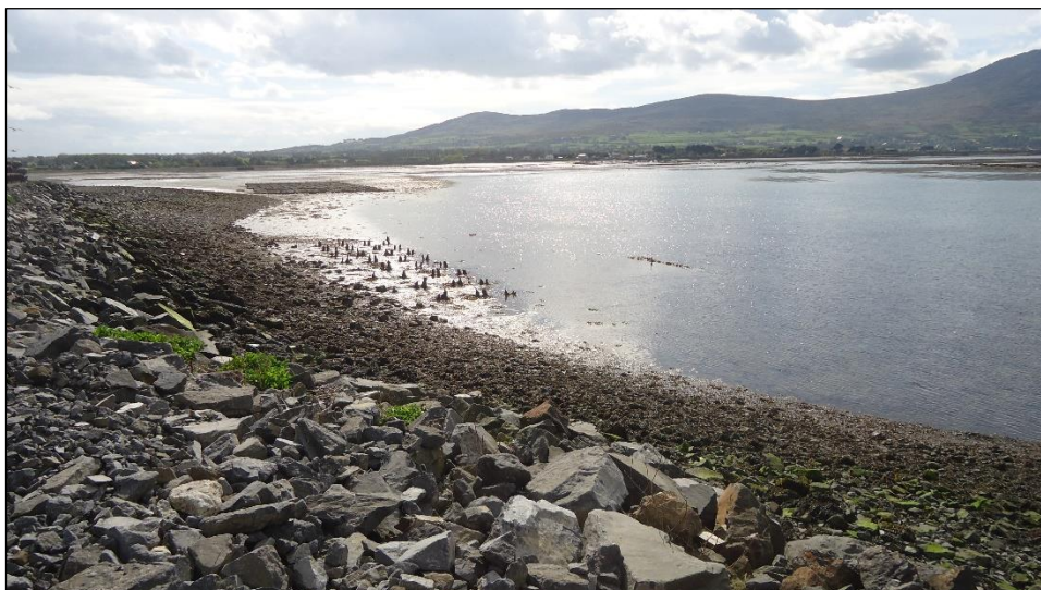
Plate 5: View looking East across intertidal foreshore at south end of the Port, showing the concrete caissons placed along the former beach area to facilitate reclamation for the Port.
