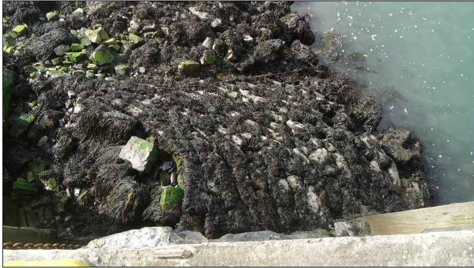
Plate 14: View looking down from quayside at the embrasure feature built in front of the stone quay at its southern end, to act as an armoured protection.
