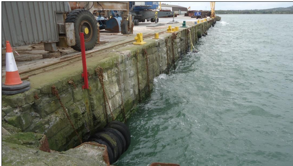
Plate 10: View from Berth 1 looking south along the façade of Berth 2.
