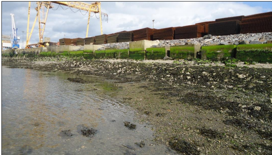
Plate 5: View looking East across intertidal foreshore at south end of the Port, showing the concrete caissons placed along the former beach area to facilitate reclamation for the Port.
