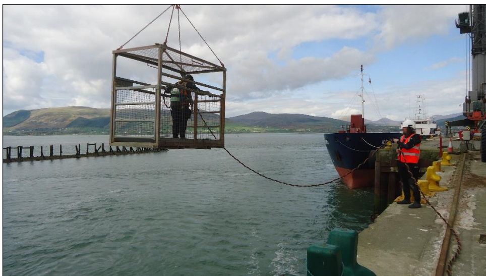
Plate 3: View showing diver being lowered in steel cage from quayside, with tender.
