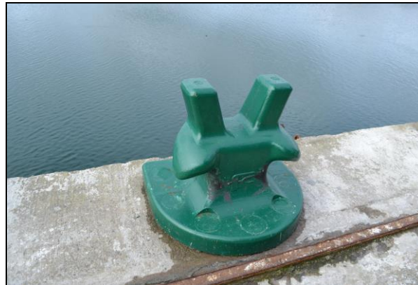
Figure 2 Typical 100tonne Bollard
