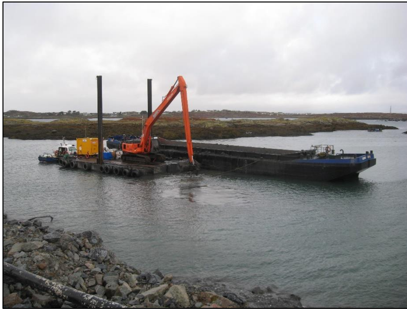
Figure 3 Typical Dredge Barge, Back Hoe Excavator, and Hopper Barge
