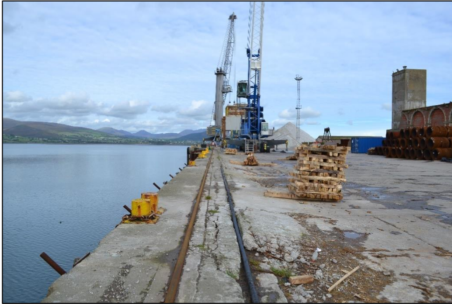
Figure 1 Deck at Berth No.2
