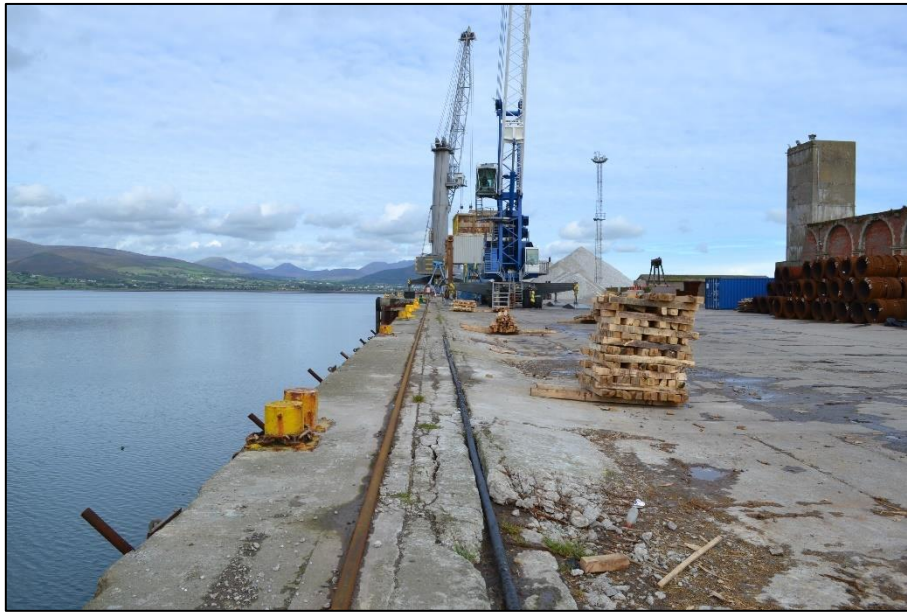
Figure 1 Deck at Berth No.2
