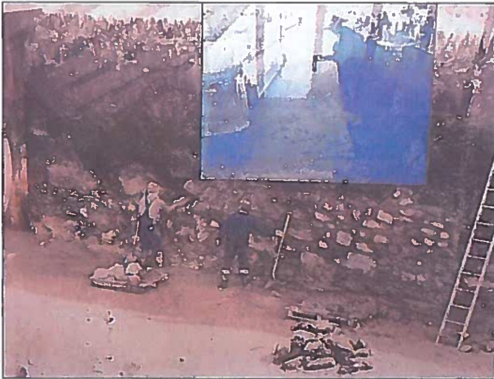
Plate 14: Detail from 1980s' photograph showing repair work to quayside stonework while the basin was drained. Source: Tara View Hotel.
