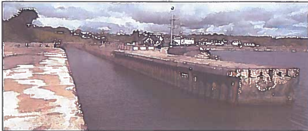
Plate 11: View looking northeast across the modern pier ends at the seaward entrance to the Harbour, showing its steel-and-concrete construction, and highlighting the weathered nature of these works.
