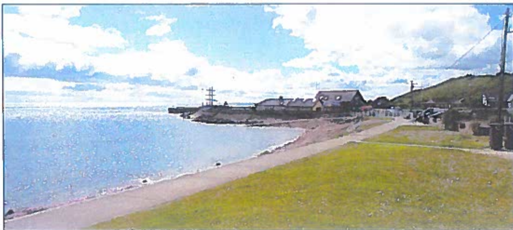
Plate 2: View looking south along spit of reclaimed land that forms the eastern side of the basin.
