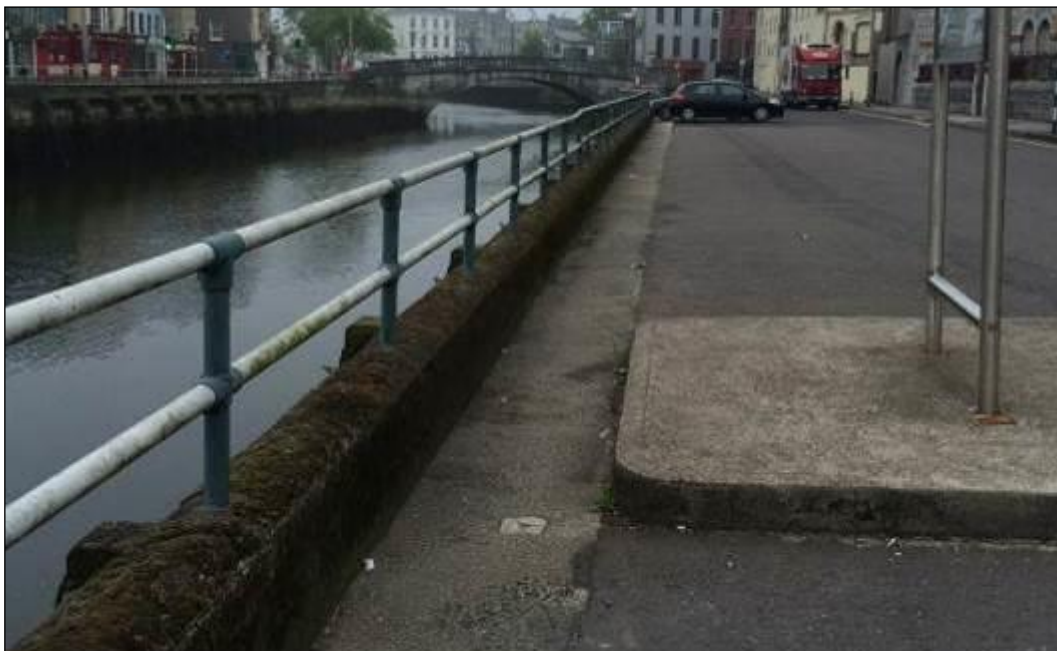
Plate 10.10: View of line of granite blocks set along top of quay walls in localised area in west half of quay, broadly opposite the Holy Trinity Church (HAN 10). This is the only section containing this stone type and may indicate localised repairs, perhaps involving inserting a heavier stone type to consolidate the underlying masonry
