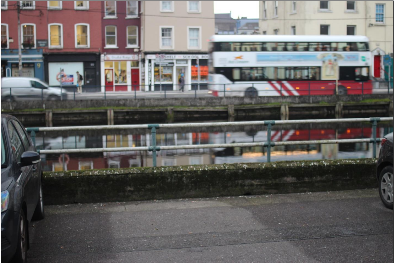
Plate 9.4: low wall and railings along Father Matthew Quay
