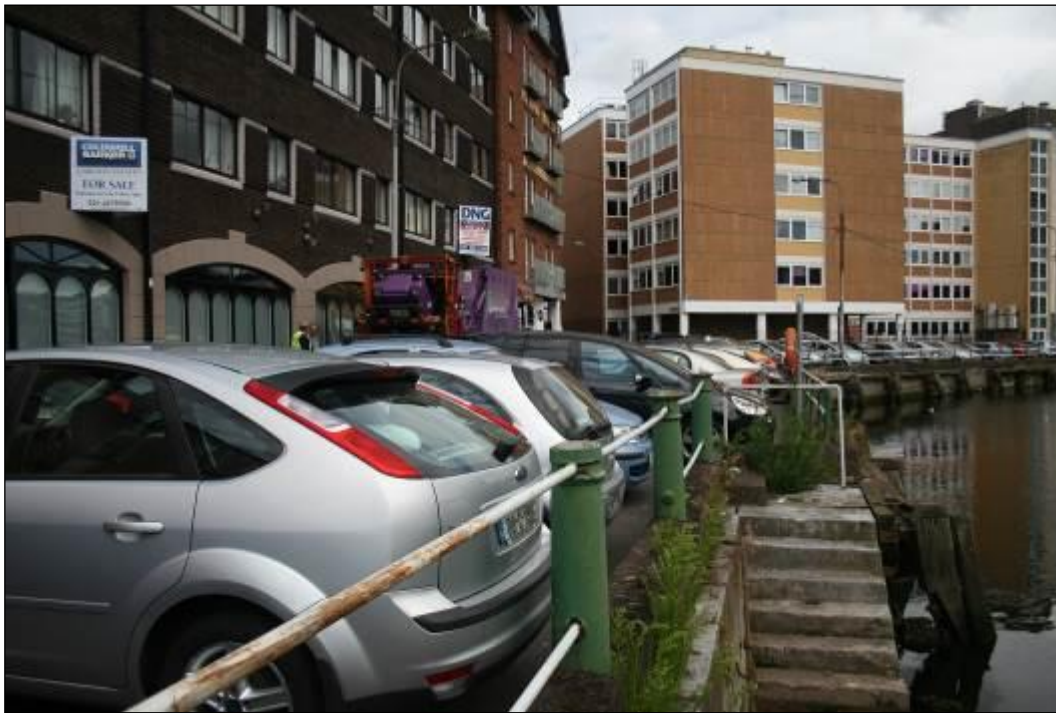
Plate 10.20: View from west towards western river steps Morrison's Quay (HAN 2) and also depicting extent of car parking adjacent to the quay side
