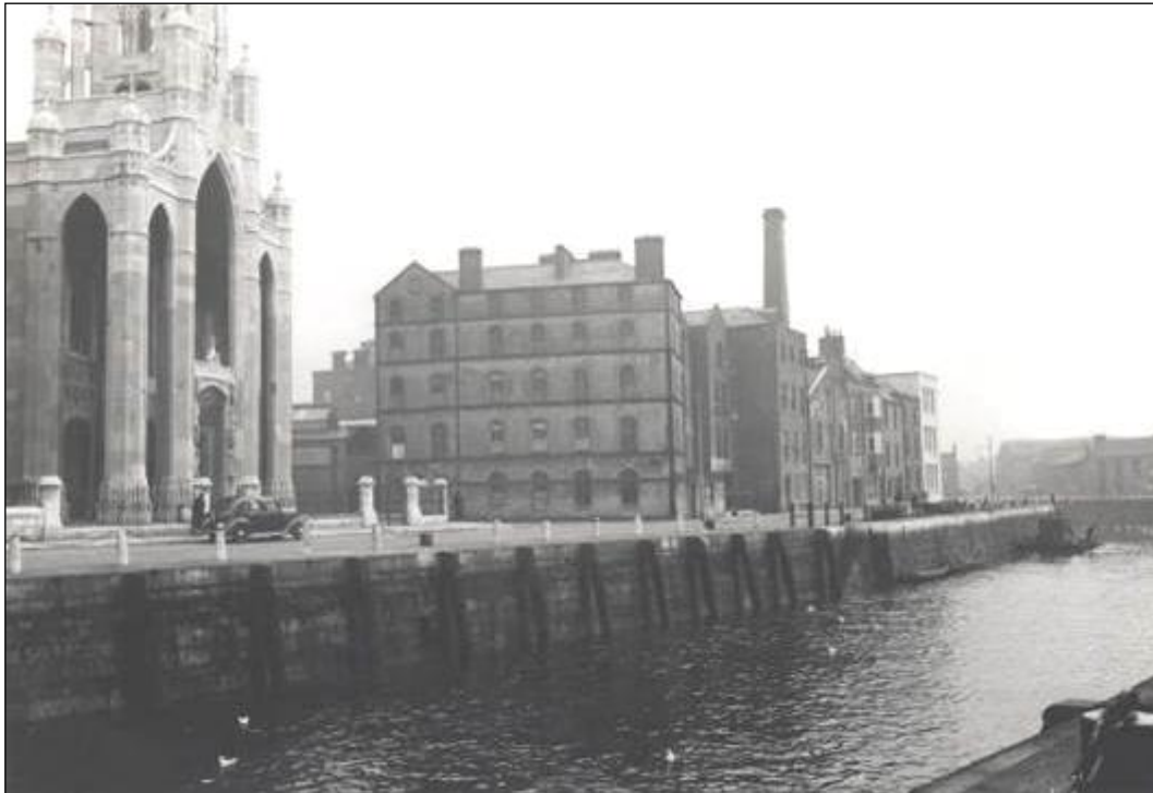
Figure 10.12: View of west end of Father Mathew Quay (HAN 1) from southwest showing the bollards and mooring posts that have been replaced by the modern railings and concrete base wall
