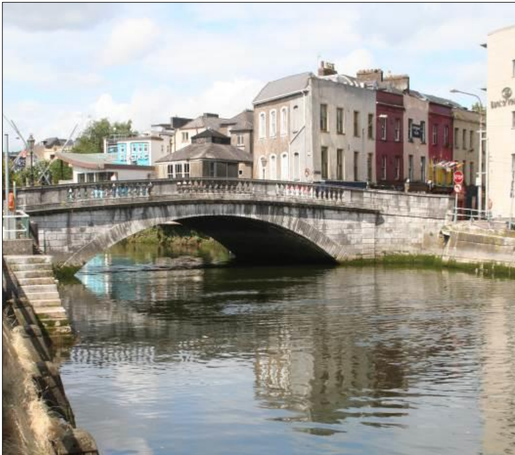
Plate 10.1: View of east elevation of Parliament Bridge (HAN 4) from George's Quay. The proposed works will involve no interventions to this structure. The intersection of the limestone ashlar quay wall at the west end of Father Mathew Quay (HAN 1) can be seen abutting the bridge structure and the wall is topped by a combination of modern railings and 19 th century bollards in this area.
