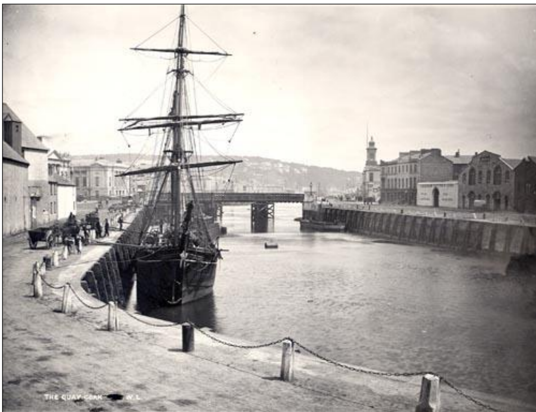
Figure 10.13: View from west of ship berthing at east end of Morrison's Quay (foreground) (HAN 2) showing bollards and chains extending along the quayside.
