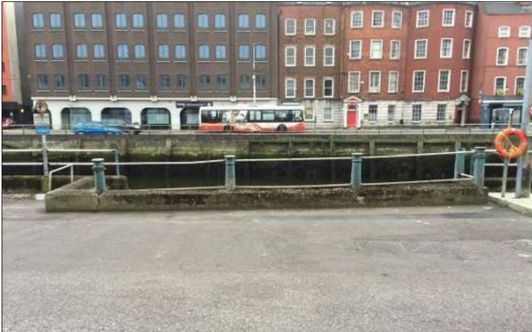
Plate 10.11: View from north of metal bollards extending around Father Matthew (HAN 1) quay steps. The steps are located opposite the area where the quay intersects with Father Mathew Street and are indicated on the 25" OSI map (1888-1913 series)
