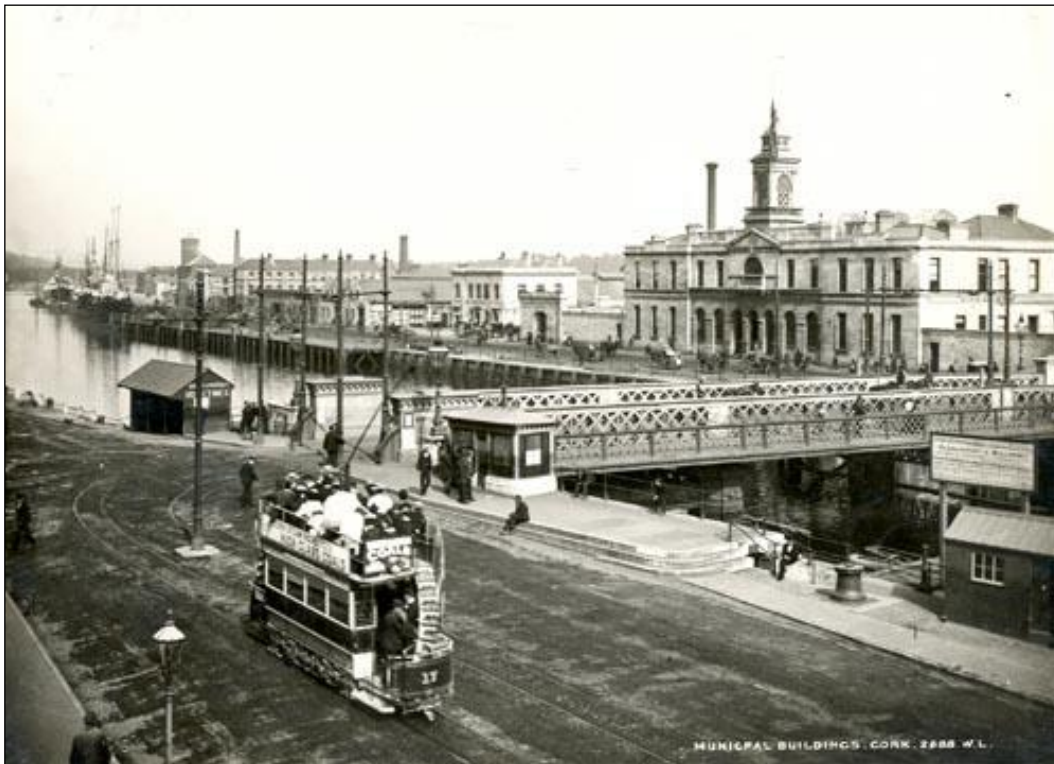
Figure 10.14: View of east end of Morrison's Quay (foreground) (HAN 2) from west showing various quayside structures and mooring posts in vicinity of the former Parnell Bridge (HAN 16) as well as the former riverside engine house (HAN 15) on the west side of the structure. The presence of an electric tram running along South Mall demonstrates that the photograph dates to the period post-1898. This area is now occupied by the modern public plaza (HAN 14) and no surface traces of the quayside features shown in the photograph remain.
