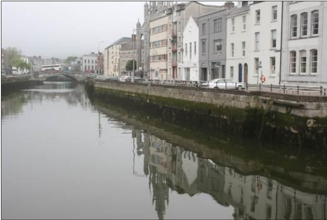
Plate 10.2: General view from east of Father Mathew Quay (taken from Trinity Bridge) (HAN 1) showing quay walls and buildings at north of the quayside
