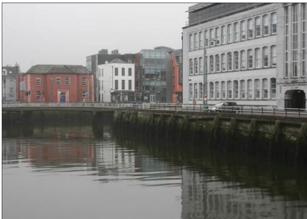
Plate 10.15: General view from east towards west end of Morrison's Quay (HAN 2) with College of Commerce (HAN 11) on right side
