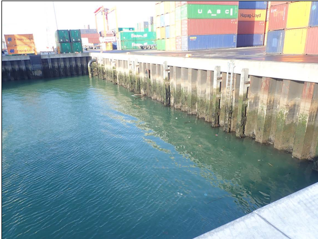
Plate 3: View looking west across north end of Berth 50 where the floating pontoon will be installed, attached to the existing Larsen piles.
