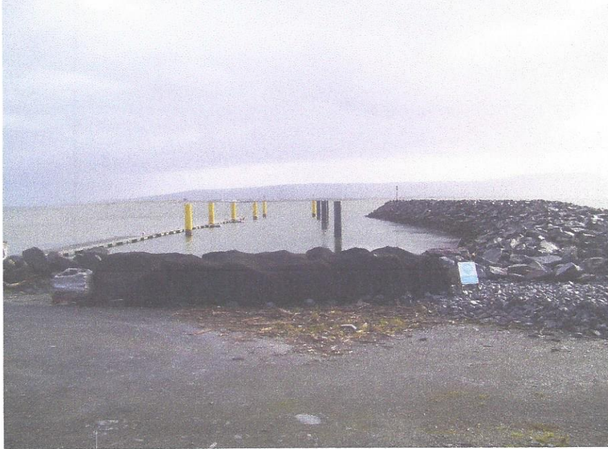
Photograph 2: Partially constructed breakwater and associated revetment works.
