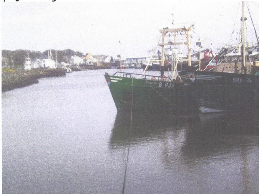
Photograph 5: Existing Harbour facilities
