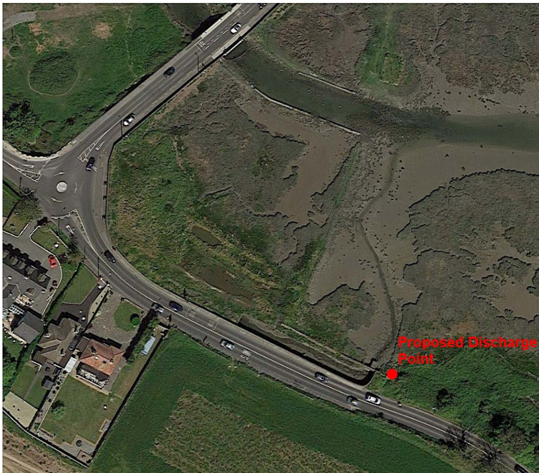
Figure 1 Photo showing location of proposed storm water outfall discharge
