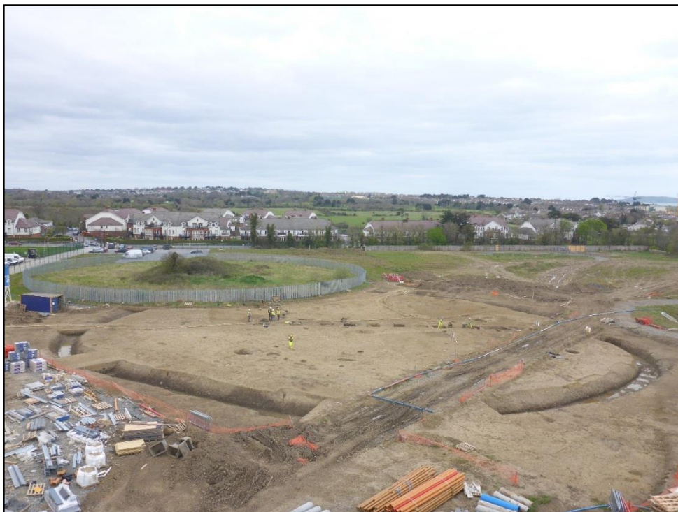
Plate 7 April 2017 –the excavation of enclosure DU015-014001 adjacent to the mound
