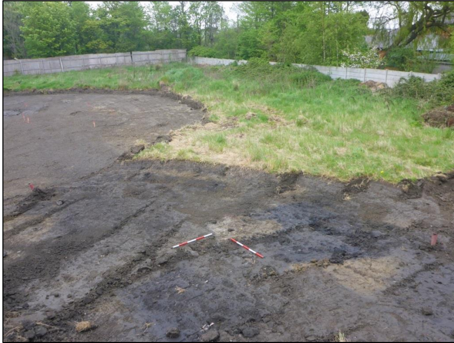
Plate 3 View to the proposed excavation area (Area 5A)
