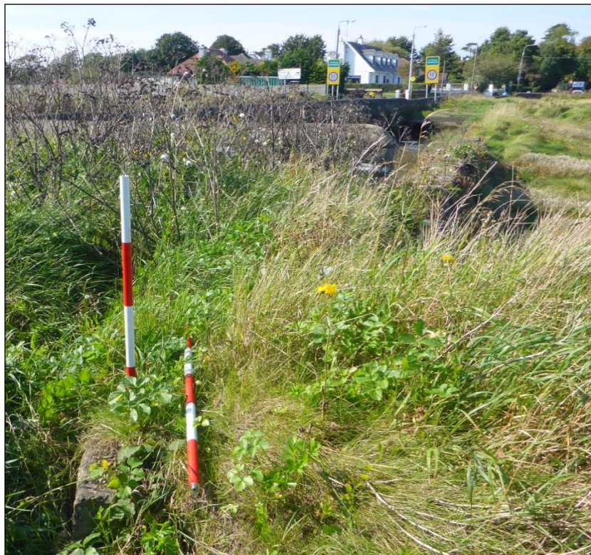
Plate 13 Rubble limestone low feature with modern inclusions, this will be breached by the proposed development
