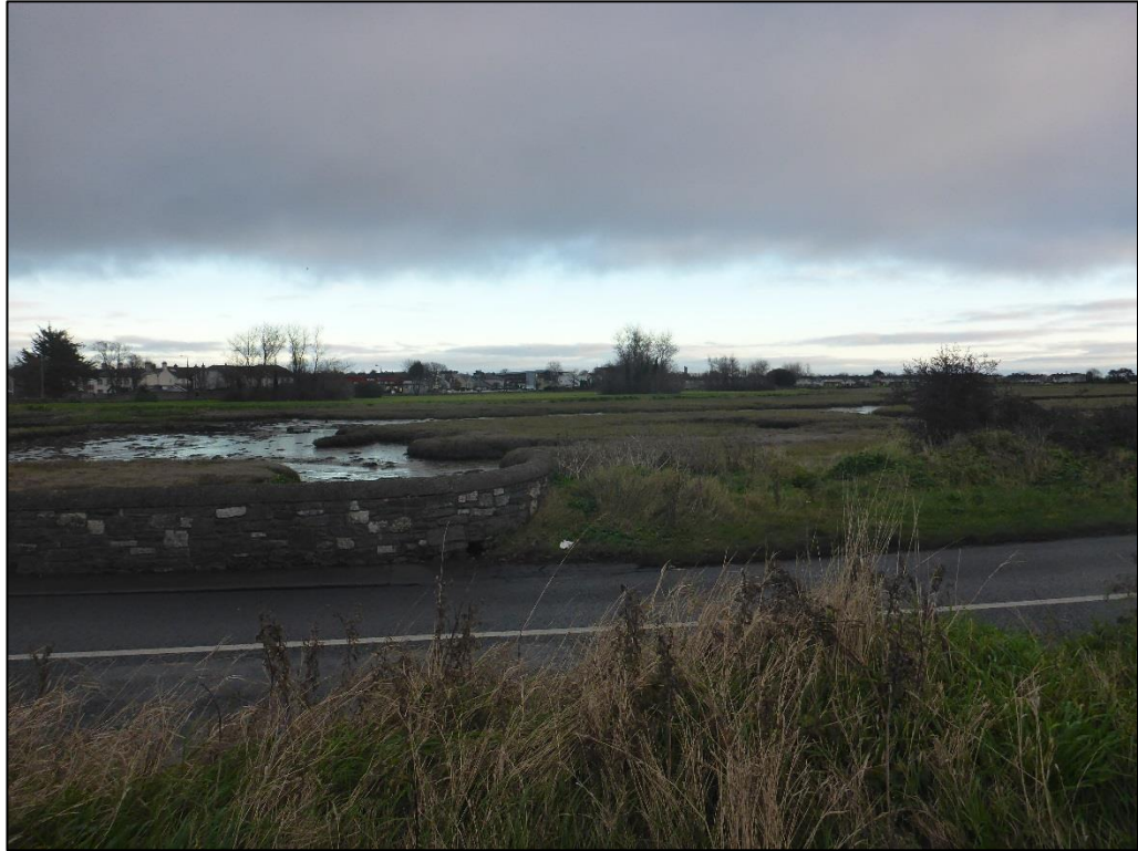
Plate 18 View to the bay from the site showing the area to be disturbed to the south of the mill race wall
