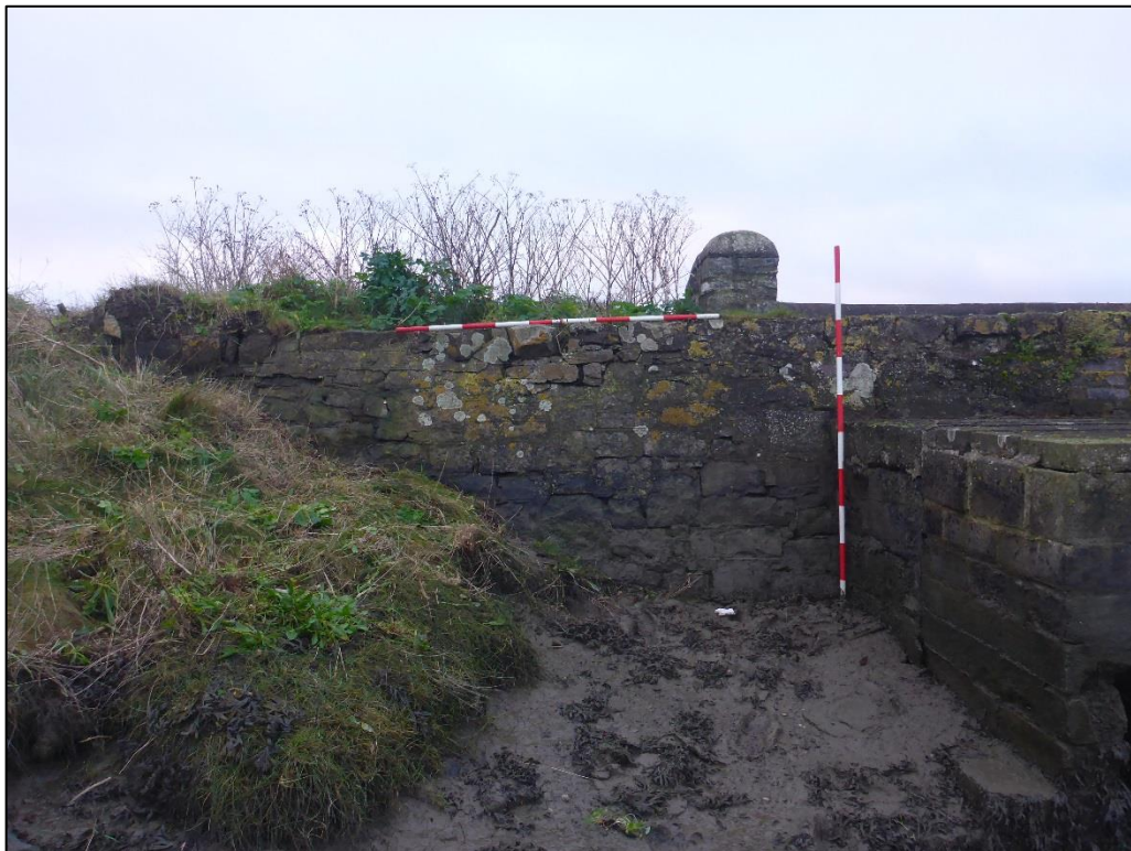
Plate 11 Roughly coursed rubble stone wall, slighted battered to the south of the culvert
