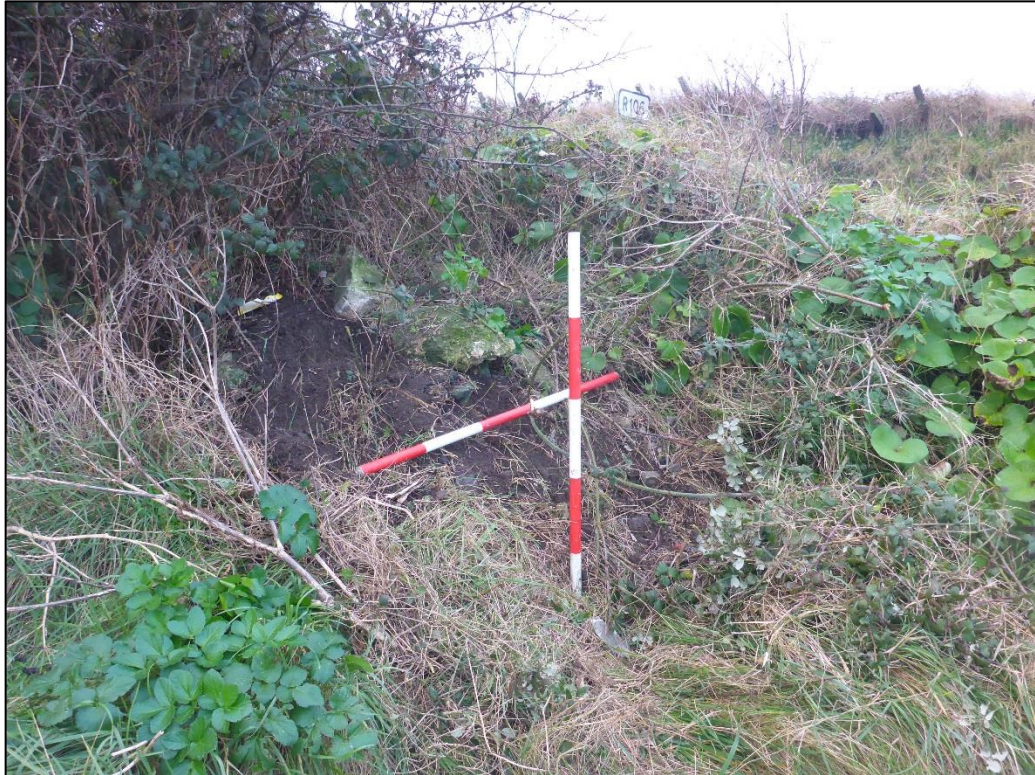
Plate 14 Concrete slab found in the undergrowth at the location of the pipe crossing
