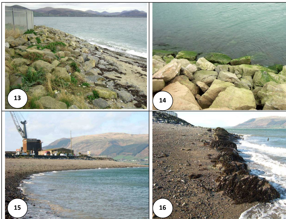
Plate 7.4: 13 = Rock armour above shore close to proposed berth; 14= Rock armour and steel palisade fencing at Greenore Point headland (HT+2hr); 15 = sand and shingle shore south of pier site (view north toward proposed ferry berth), 16 = lower shore at low spring tide (7-3-12) showing gravelly sand shore with line of boulders just at the site of the proposed berth.
