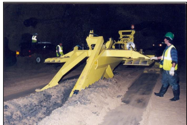
Figure 2. Typical Plough Installation
