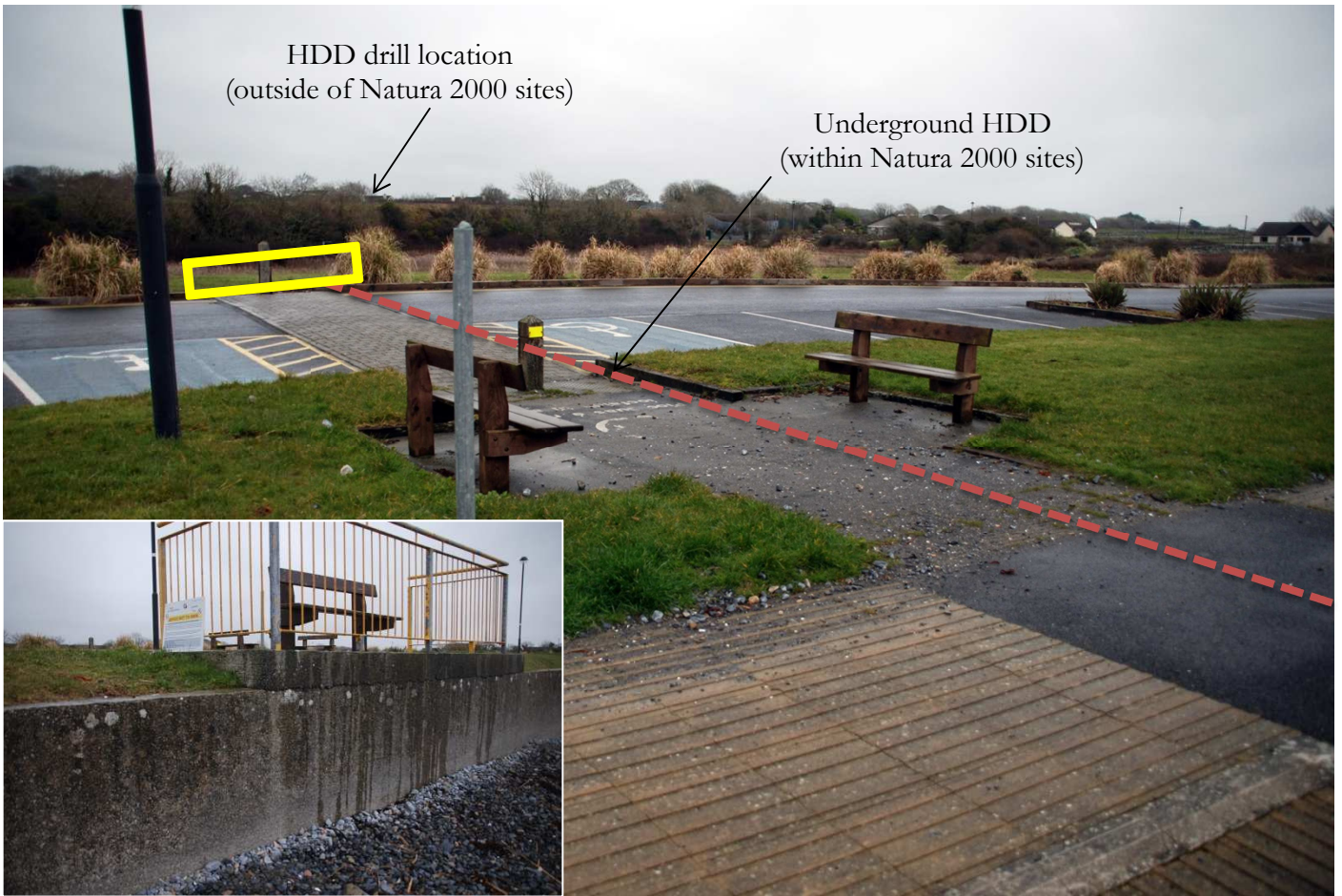
Plate 7: Site of HDD drill set-up
