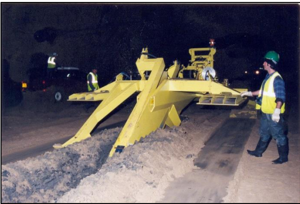
Figure 27. Typical Plough Installation.
