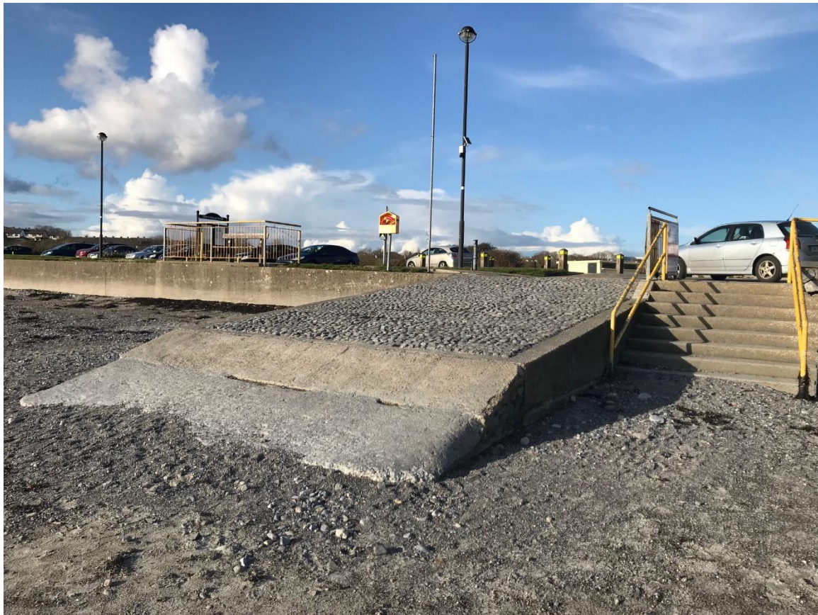
Figure 28. Foreshore Access Slipway.
