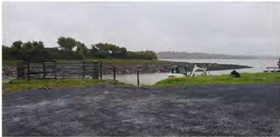
Plate 3: Pier and top of slipway. Looking SE
