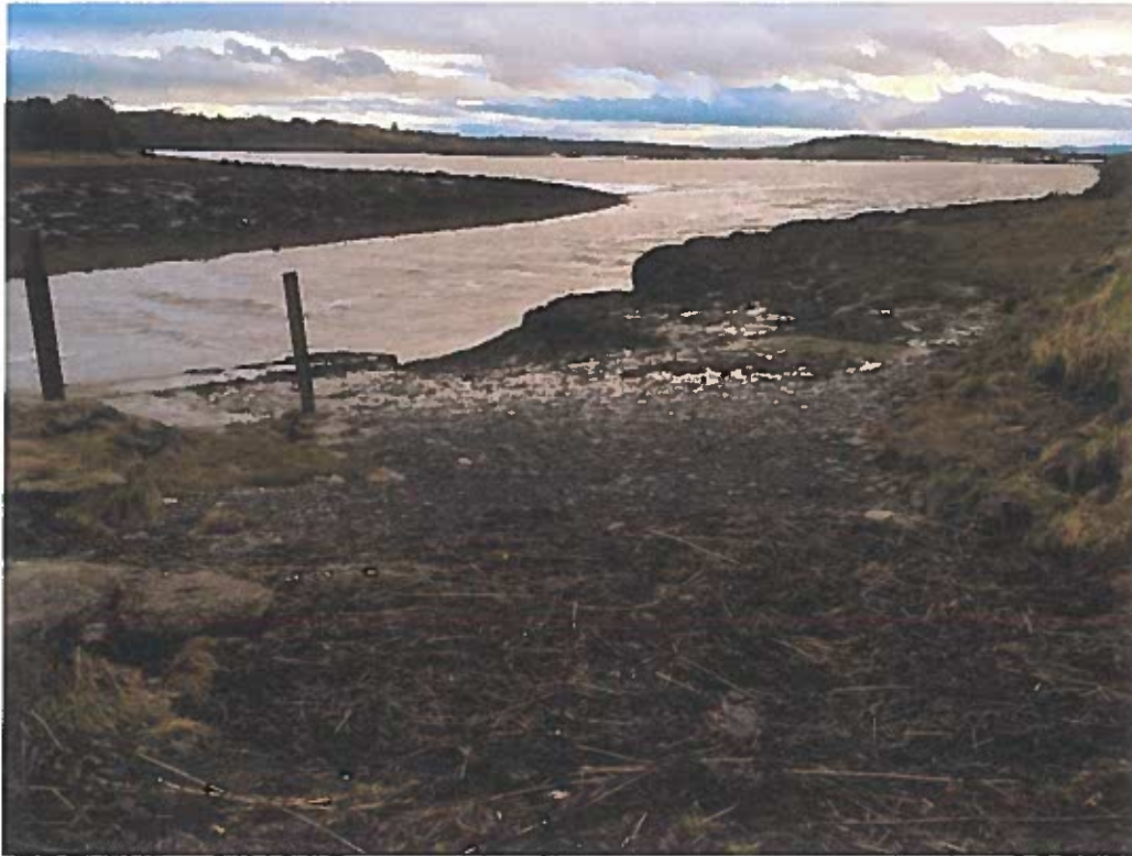
Views of existing slipway adjacent to quay at Crovraghan (December 2017)
