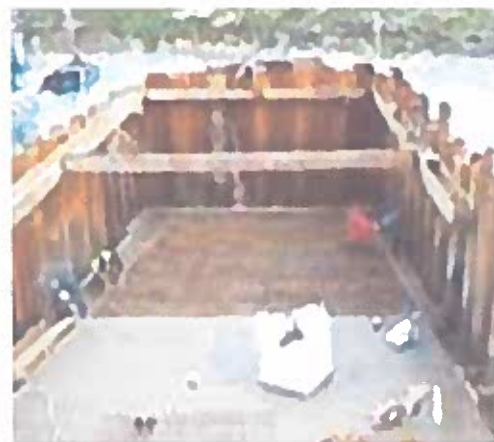
Figure 1; Typical shuttered area for slipway construction
