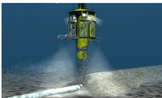
Figure C5 – Rock placement along exposed pipeline
