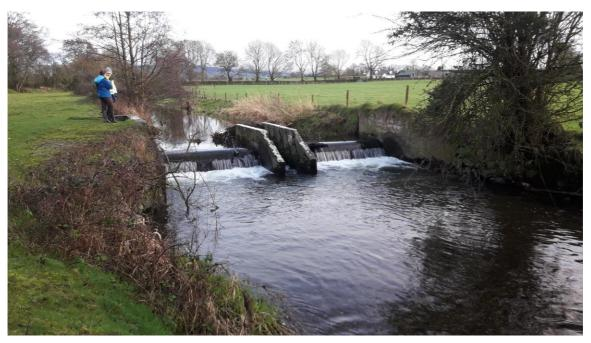
Figure 4.2. Gravel trap on the Ollatrim River, in the Nenagh catchment.
