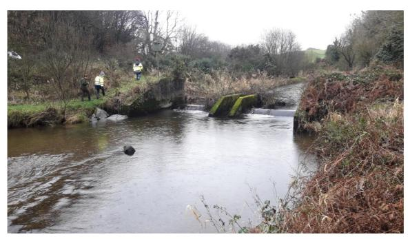
Figure 4.1. Gravel trap on the main stem of the Nenagh River.
