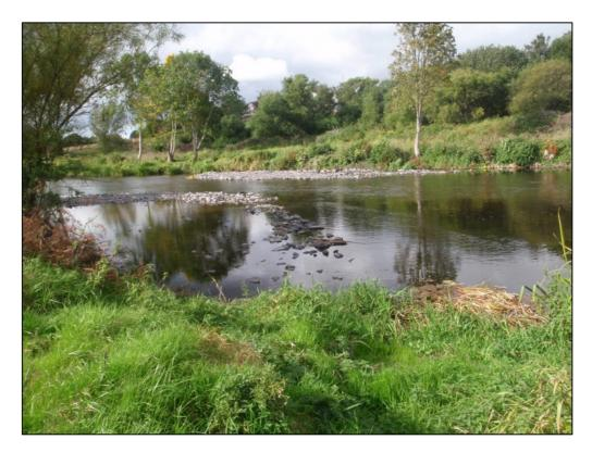
Figure 2.4. Paired deflector on the Boyne main channel (C1).
