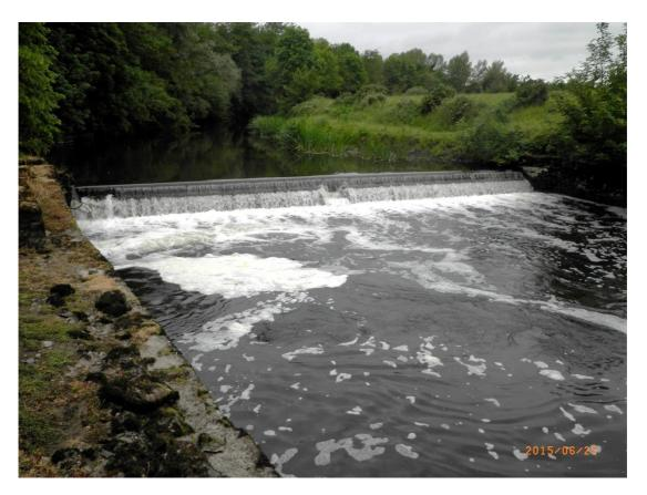
Figure 5.4. Martry Mill on the Kells Blackwater (Boyne CDS) a structure highlighted for mitigation (rock ramp). This is a high impact barrier to adult salmon and a complete barrier to lamprey.
