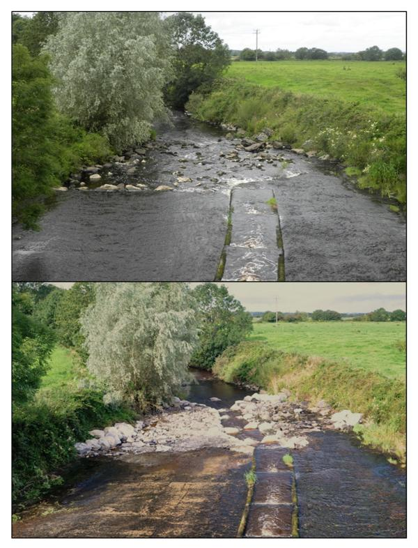
Figure 5.3. 2015 remediation works at Ahavoher Bridge on the Galey River (Feale CDS), Pre (top) and Post (Bottom) works.
