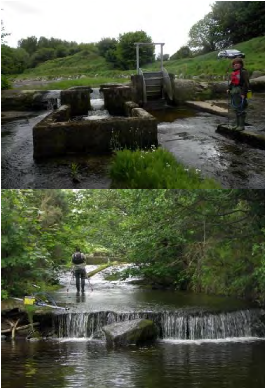
Figure 6.1. Cadamstown Sand Trap on the Kilcormac Silver (Brosna Tributary: C3(1)), Fish pass (top) and downstream end of structure (Bottom) showing drop and long concrete sill.
