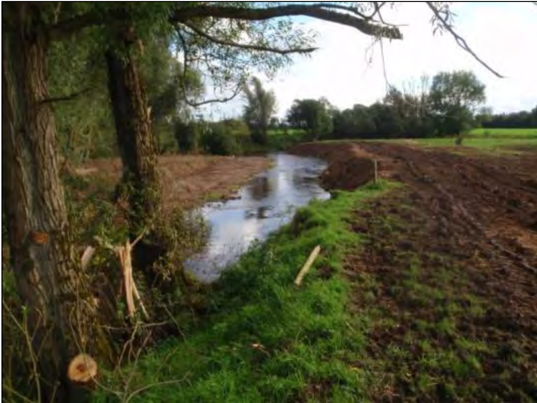
Figure 2.6. Berm management and bank protection work Loobagh R. post works.
