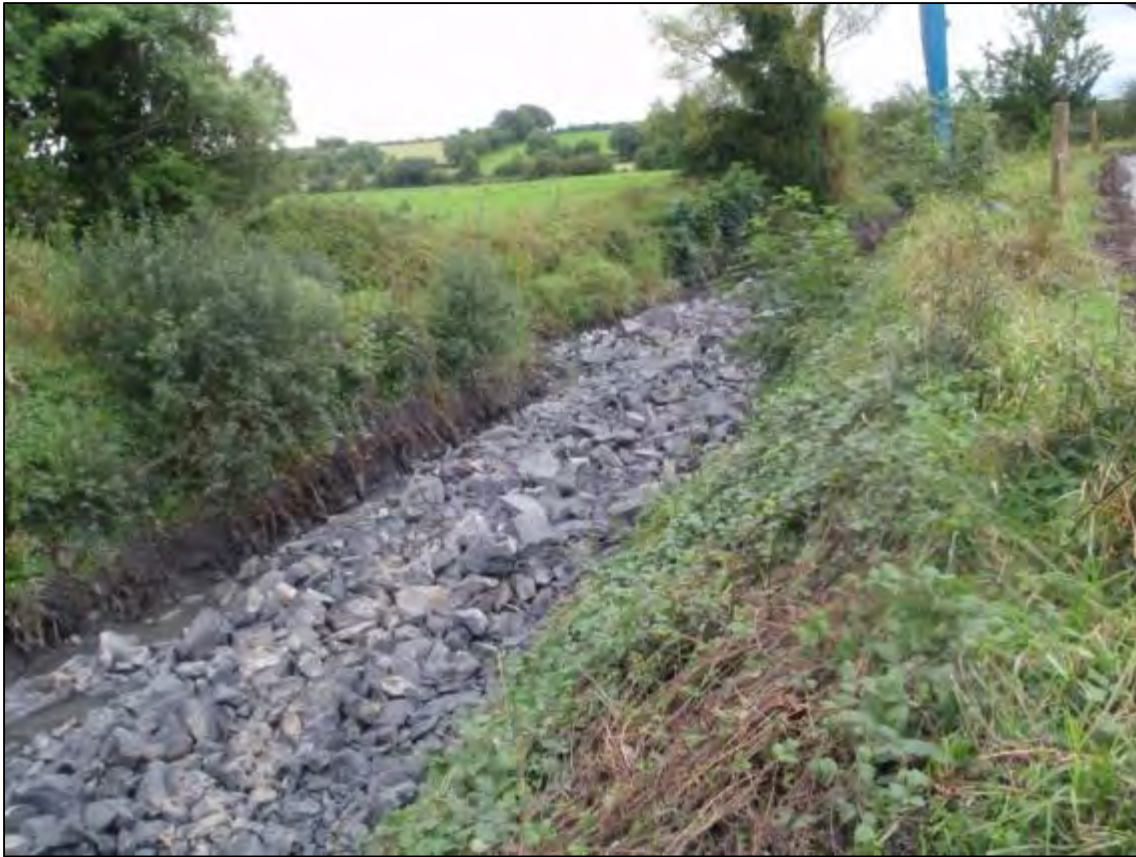
Figure 2.4. Rock breaker working on the Kilcrow R. Ballycahill Bridge.
