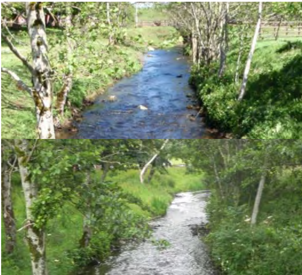
Figure 4.5. Constructed in 2015 Experimental Site 1 consists of two paired deflectors with pools and gravel shoals (Top Pre works: 2014, Bottom Post works: 2016).
