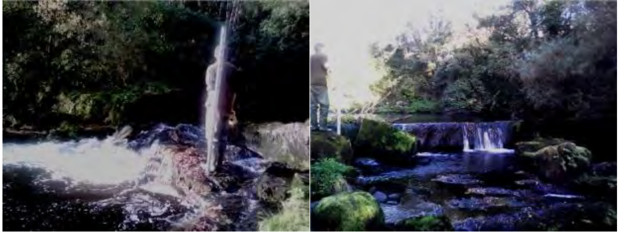
Figure 4.21. Man-made barriers on the Owenmore River, comprising of natural rock outcropping augment with concrete, surveyed October 2016.
