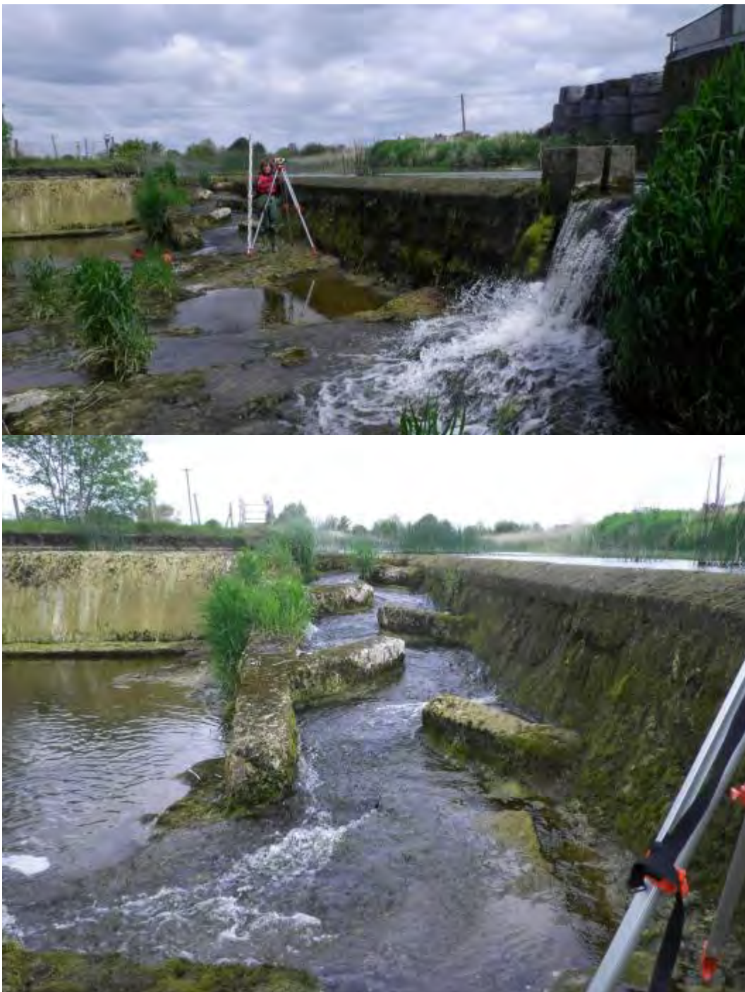
Figure 6.2. Fish passage options at Ballycahill Weir (25/5/2016), overflow sluice top, fish pass bottom.
