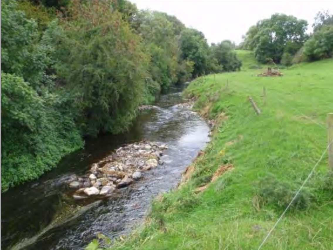
Figure 2.3. Gravel shoal at tail of pool with paired deflector Dee River.
