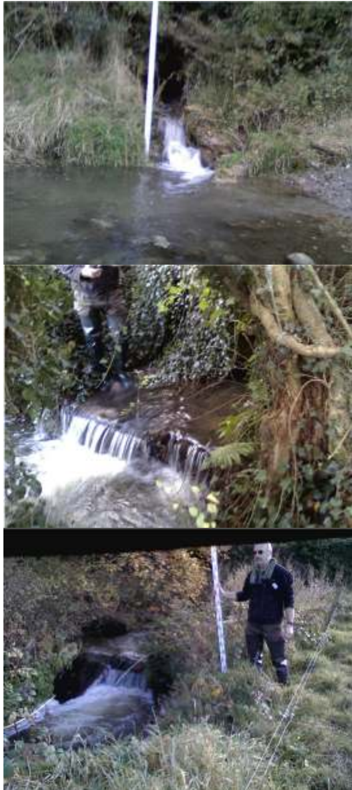
Figure 3.4., 3.5. & 3.6. Some of the barriers surveyed in the Southern Inny Basin during 2017. (Fig. 3.4 C37 (culvert & ford), Fig. 3.5 C8/8 (bridge apron), Fig. 3.6 C18 (barrier displaying a weir face & vertical drop))
