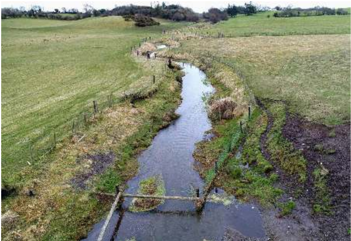
Figure 2.13. Site 3 looking downstream in January 2018, showing extent of instream vegetation dieback during winter months, top of Study Site 3 at cattle drink see figure 2.15
