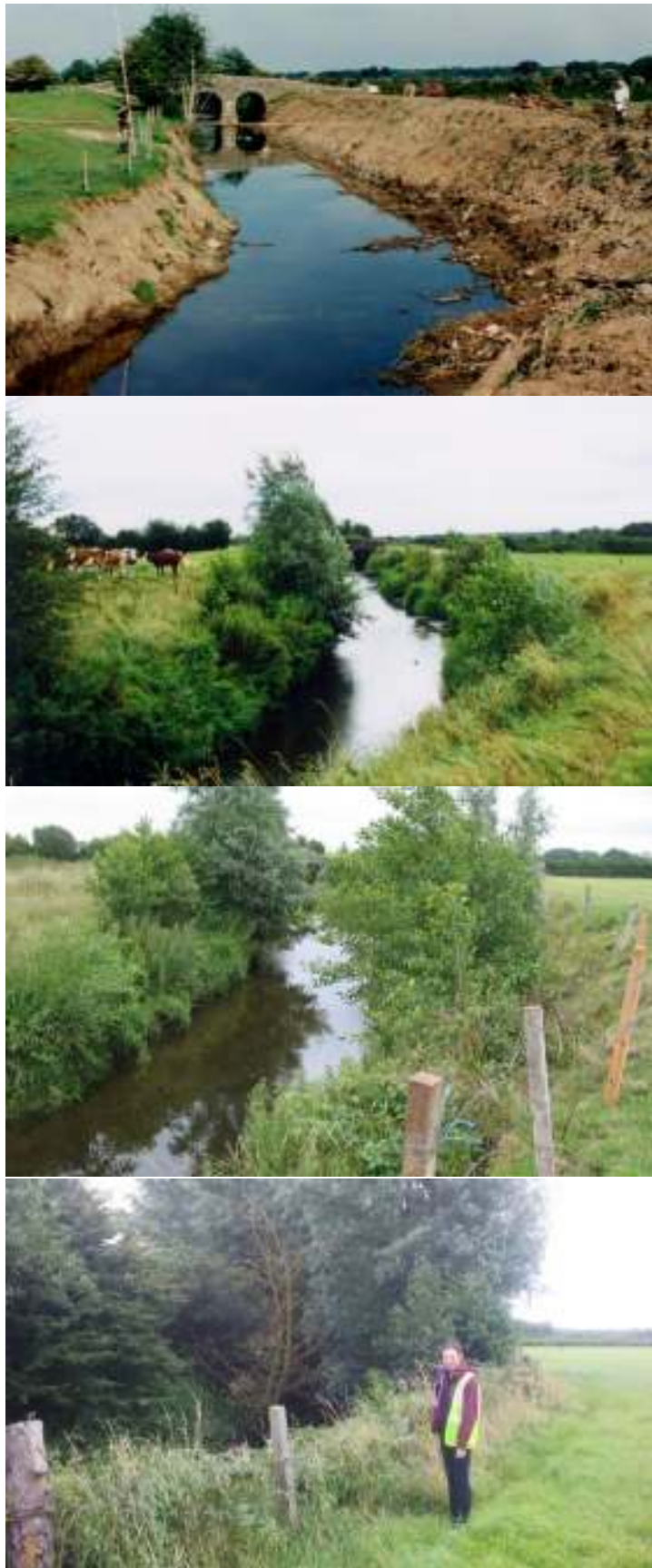
Figure 2.26. Site 4 (Chg 119) on the Clodiagh downstream of Annomoe Bridge, top to bottom: immediately post maintenance 1996, 2002, 2004 and 2017
