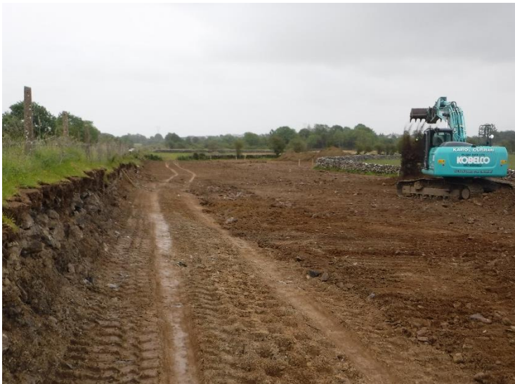
Figure 3a & 3b; Second Stage Channel Formation & Embankment Construction
