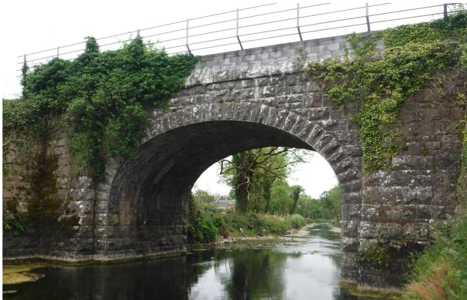
Figure 4; UB154 Railway Bridge
