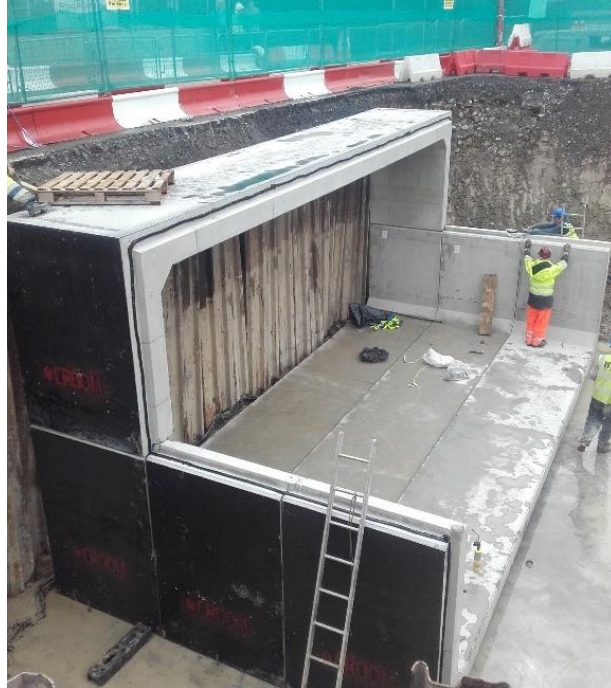
Figure 2; Culvert Installation
