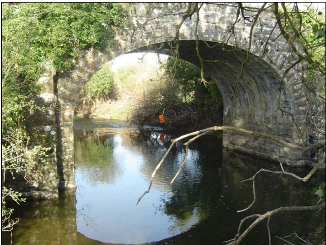
Photo No. 5 Railway Bridge looking downstream through the stone arch.
