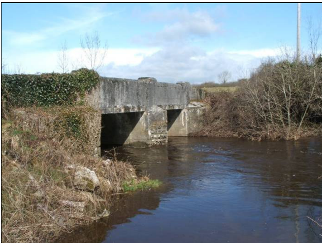
Photograph No. 8 Rinn Bridge taken from the upstream left bank
