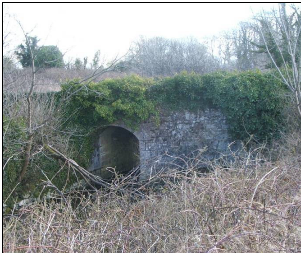
Photograph No. 15 Downstream face of the Aggard Bridge
