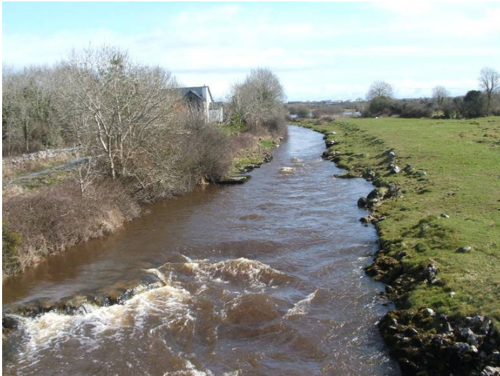
Photograph No. 16 Typical section of “canalised” channel along the Dunkellin River
