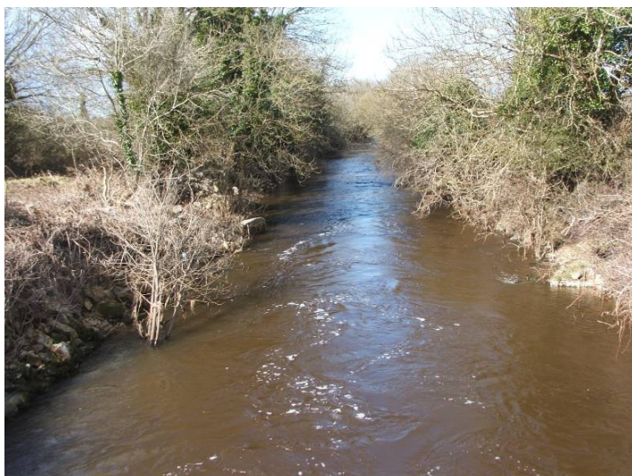
Photograph No. 17 Typical overgrowth along the Left and Right Banks of the Dunkellin River
