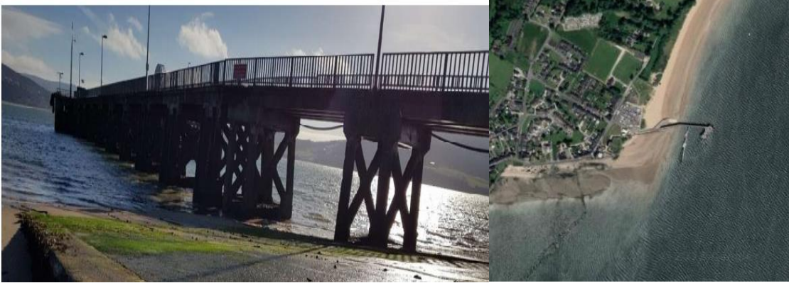
Figure 1 Image of viaduct from 2021 Condition Report; Google Maps (2023)
