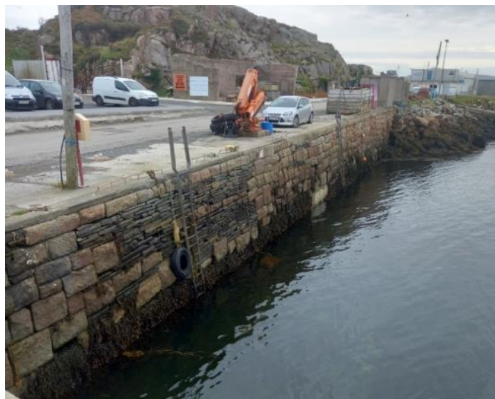
Figure 1 The current pier and location (from application documents).
