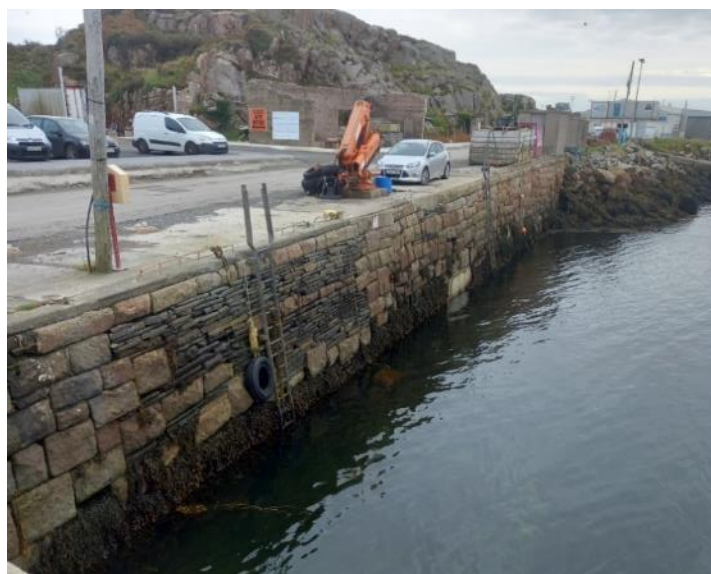
Figure 2-1. The current pier and location
