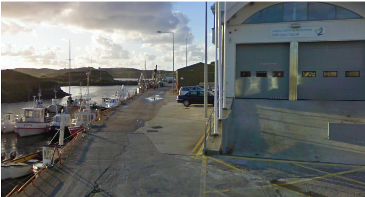
Figure 1.2. Google streetview imagery of Bunbeg pier
