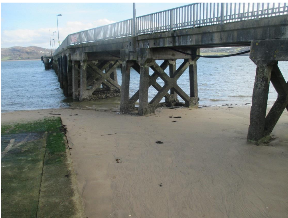
Photo 2 – View of viaduct from shore end.
