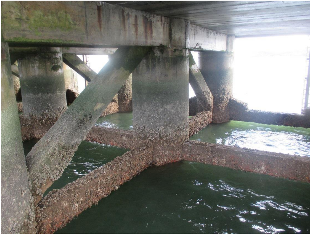
Photo 5 – Typical pier head frame arrangement.
