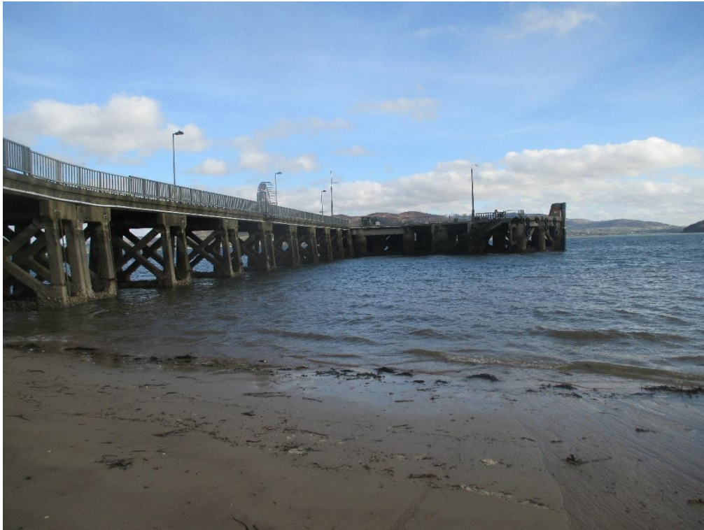
Photo 1 – General view of pier.
