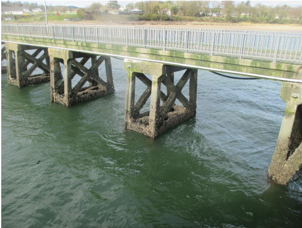
Photo 3 – View of viaduct from pier head.
