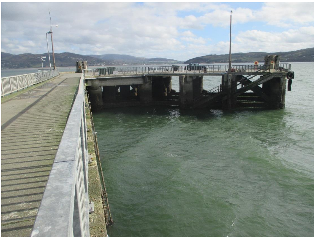
Photo 4 – View of pier head from viaduct.
