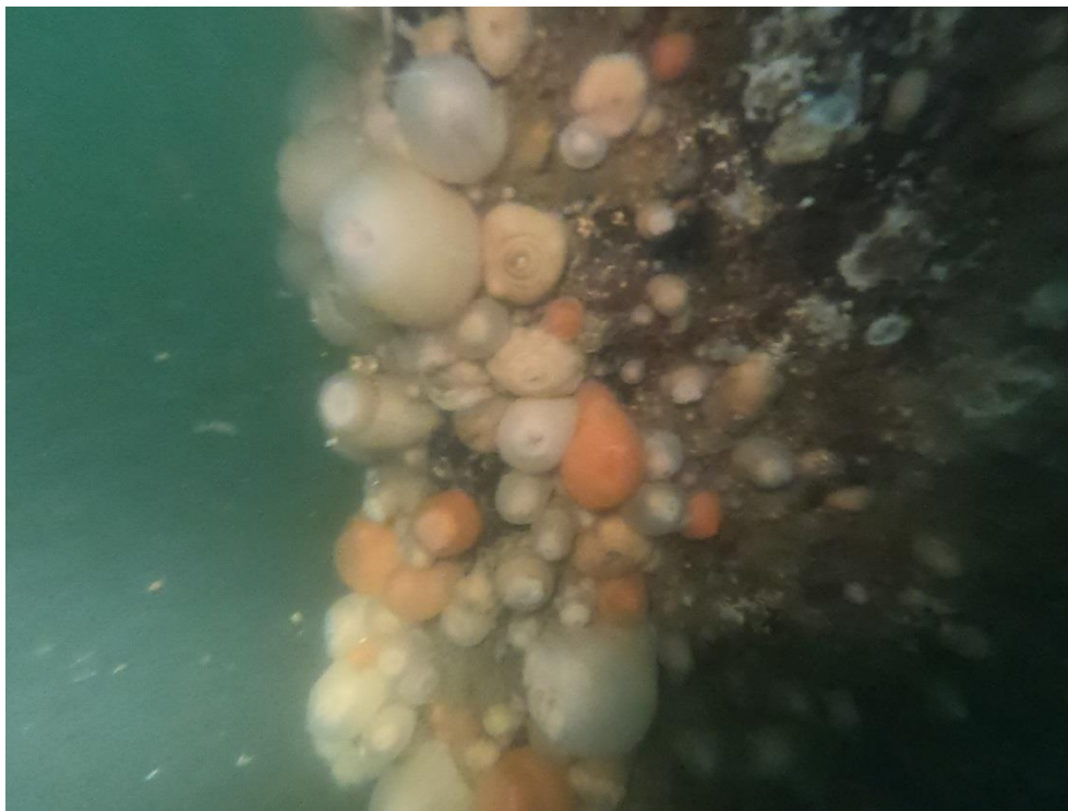
Fig B8 - Viaduct Column – Typical Condition
