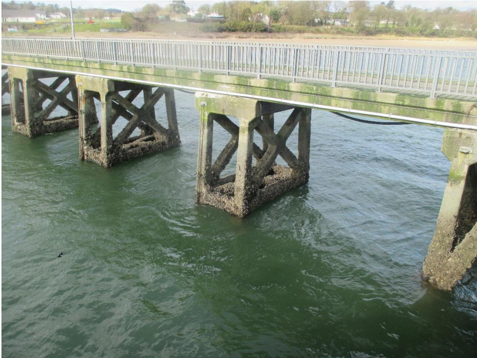
Fig B3 – View of Viaduct from Pier Head – Typical Frame arrangement
