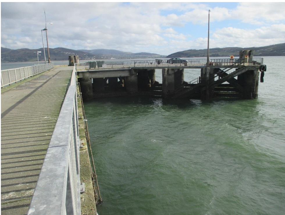
Fig B4 – View of Pier Head from Viaduct
