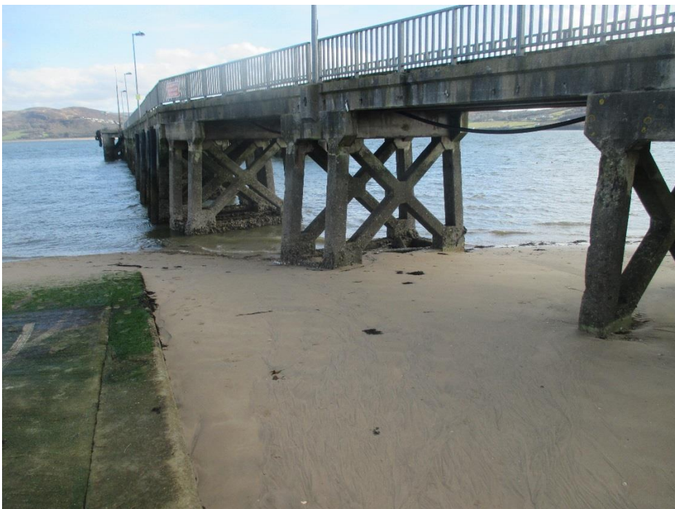
Fig B2 – View of Viaduct from Shore end.
