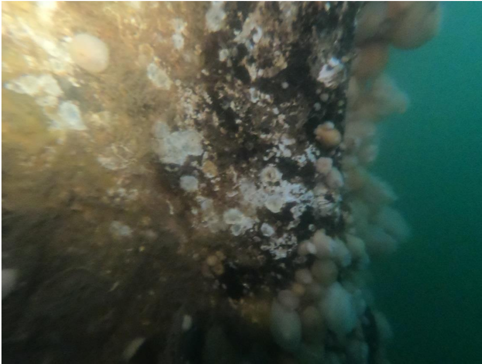
Fig B9 - Typical Concrete Condition
