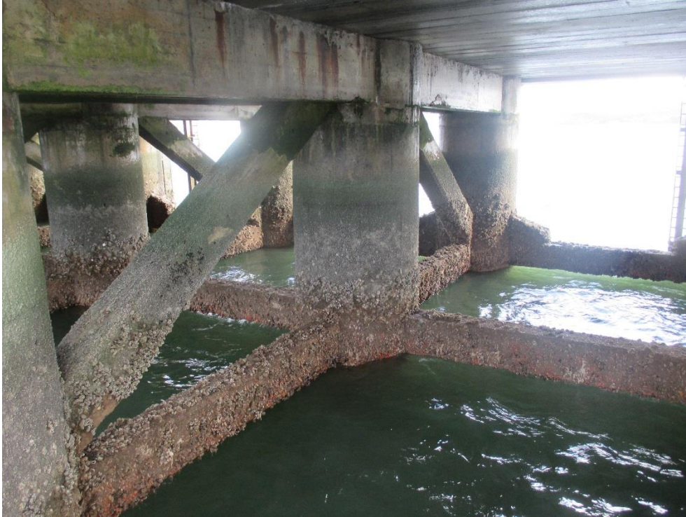
Fig B5 – Typical Pier Head Frame Arrangement
