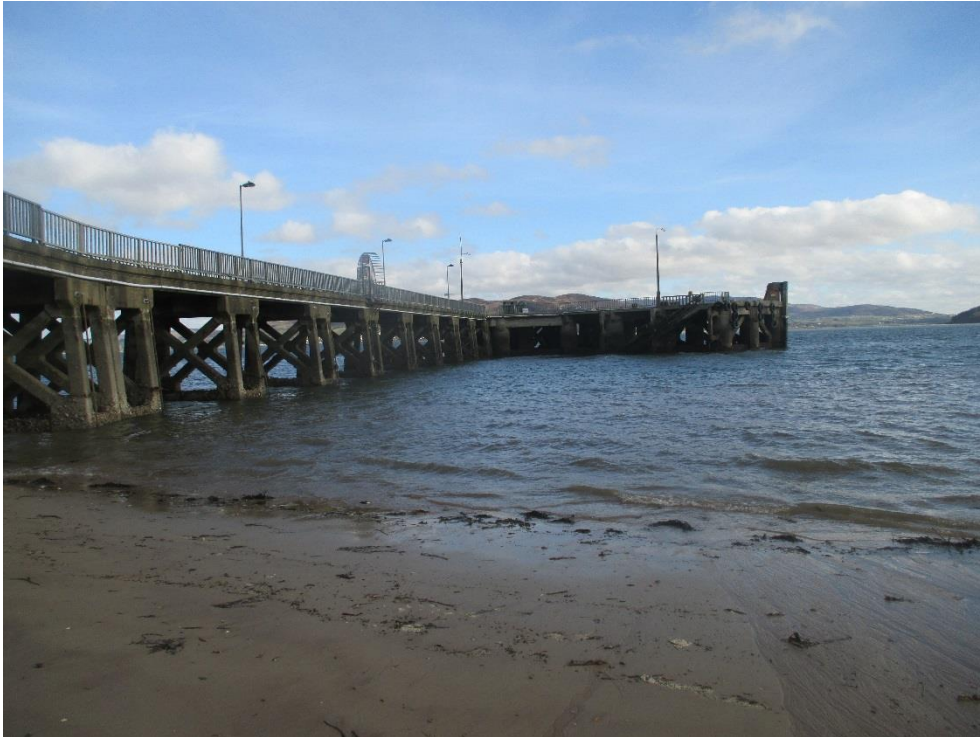
Fig B1 – General View of Pier
