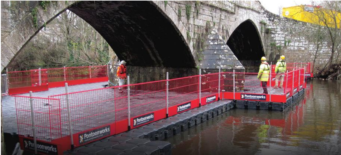
Figure 3. Example of working platform (image courtesy of Donegal County Council).
