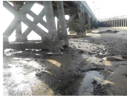
Plate 2. Looking east from under /beside the pier to the south.
