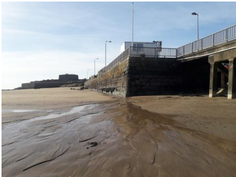
Plate 3. Looking west, southern side of the pier looking towards the village.
