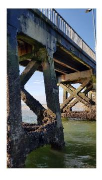
The lower beams and the diagonal cross bracings in the horizontal plane are in good condition.
