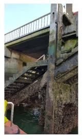
The beams supporting the deck are in need of repair to varying degrees. Some beams will require patch repair over a limited area whilst other beams will require a full depth repair over the length of the soffit with additional patch repairs on the sides. The level of deterioration has increased but not as significantly as the Viaduct section since the 2008 report.
