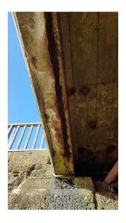
There are large areas of concrete spalling and in several the beams reinforcement is exposed. In some areas where the concrete has spalled away the reinforcement is severely corroded.
