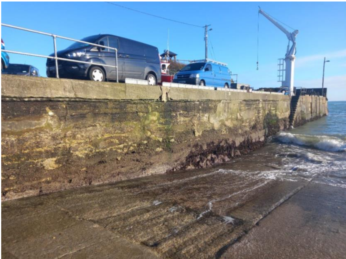
Figure 3.1. Existing quay wall
