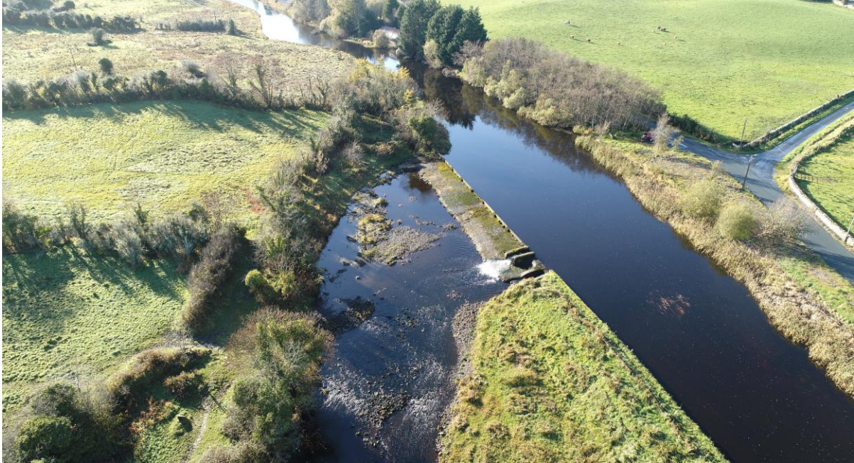
Figure 2.22 Oblique drone picture of Stewart's weir, on the Boyle River.
