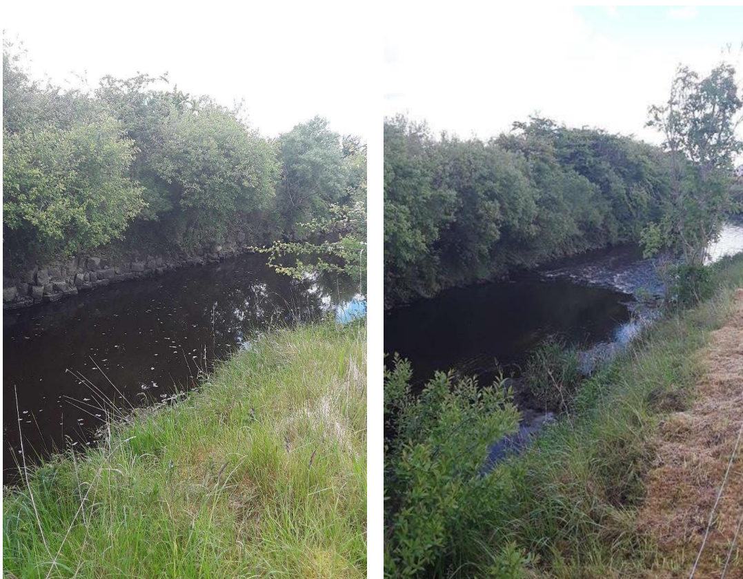
Figure 2.13 Reinforcement along the bank (left) and weedkiller used along the bank top (right) on the main Lung (C1).
