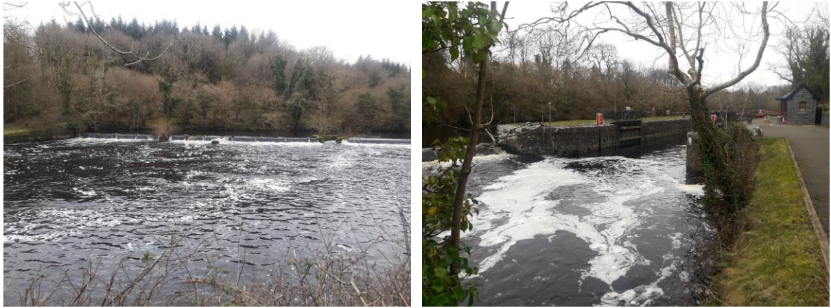
Figure 2.20 Knockvicar weir (left) and lock gate (right) on the Boyle River.
