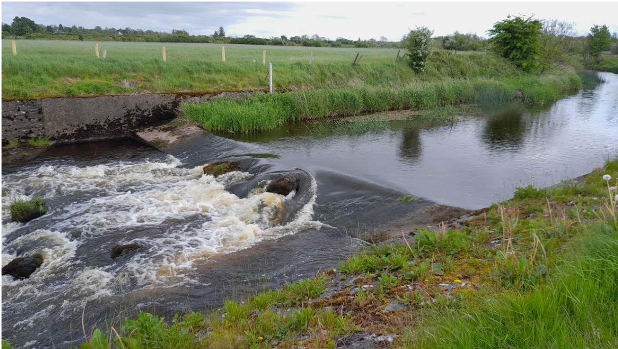
Figure 2.23 Weir on the Lung River at Ballaghadeerreen.
