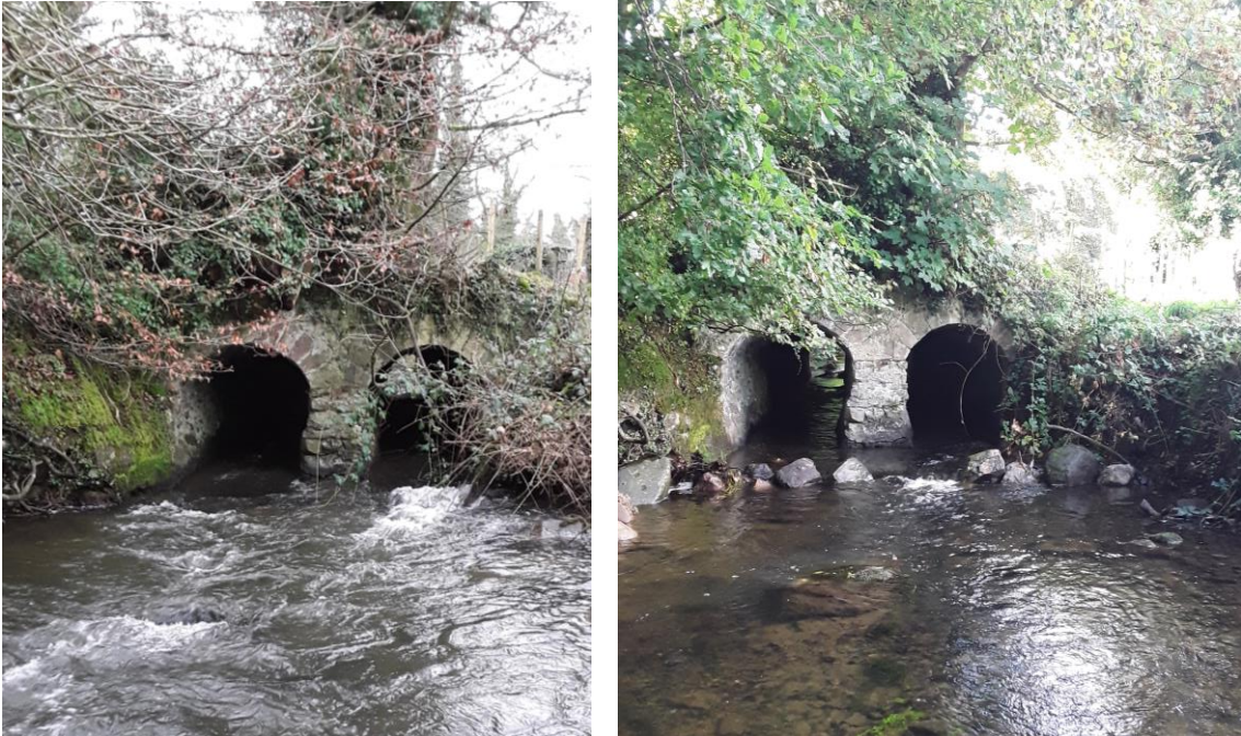
Figure 4.9 Strategic positioning of boulders at a bridge apron to alleviate a minor drop (right). Note that the photo on the right is taken during very low water levels.
