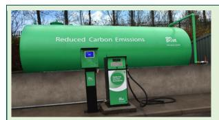
In September 2021, An Post was the first company to roll out a trial of Hydrotreated Vegetable Oil fuel (HVO), which is over 90% less CO<sub>2</sub> intensive than fossil diesel. An Post retrofitted an existing 45,000 litre tank and diesel pump, engaging with the Circular Economy by reusing an existing tank instead of buying new.
