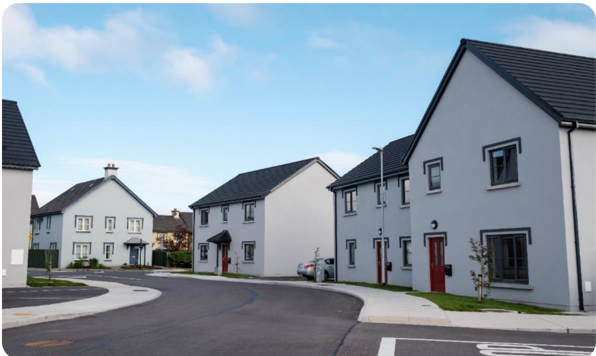
Barraduff, Killarney, Co. Kerry delivered by Co-Operative Housing Ireland
