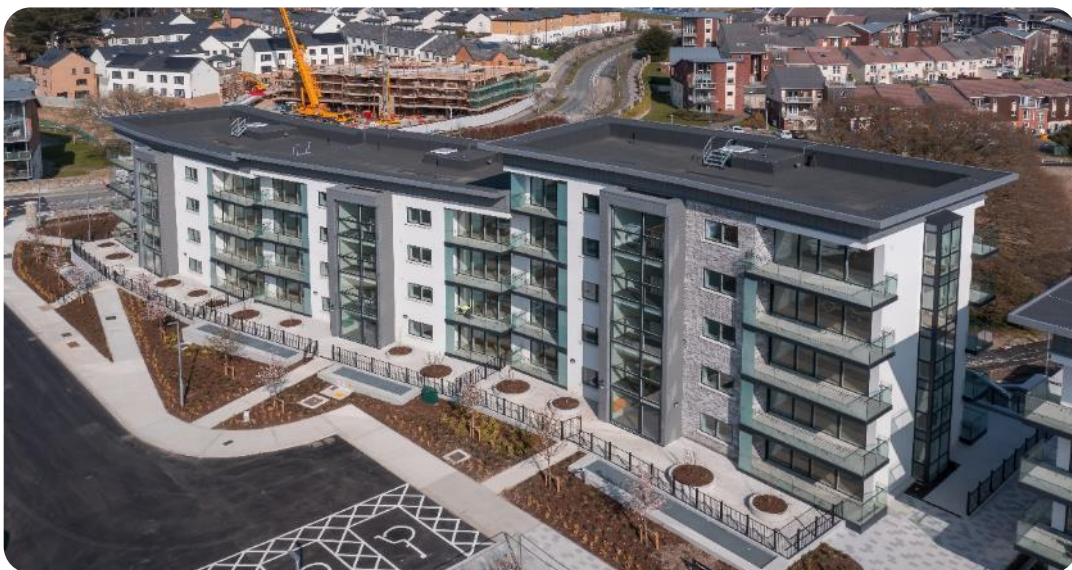
Woodstown, Enniskerry Road, Stepside delivered by Tuath Housing and Respond
