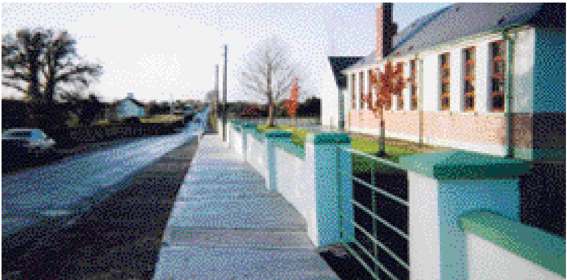
Above: Dunkerrin NS, Dunkerrin, Co. Offaly – Painting of exterior wall and gates
