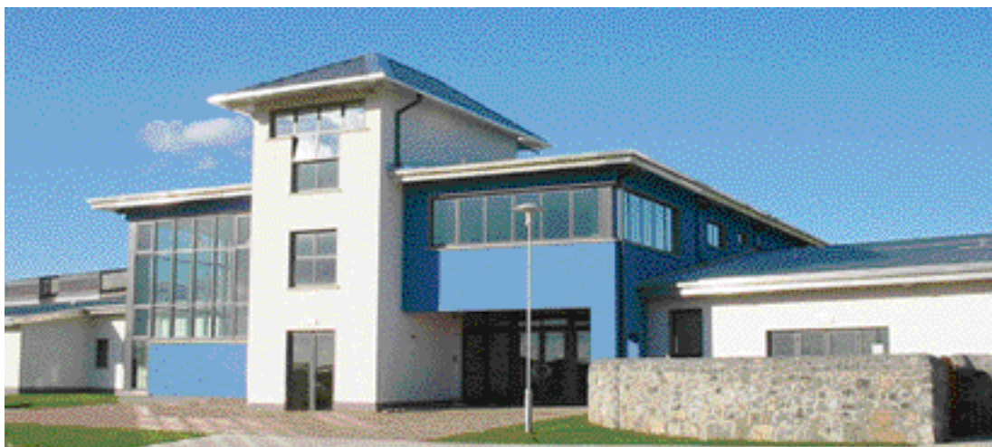
Above: St. Attracta's Community School, Tubbercurry, Sligo – built as a PPP project in 2002
