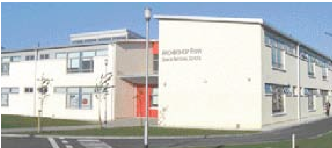
Above: GRD project at Archbishop Ryan National School, Balgaddy, Co. Dublin – completed in 2005
