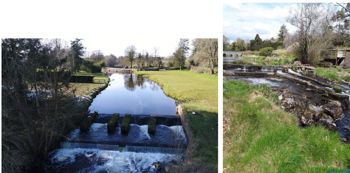
Figure 2.27 The stepped weirs at Mahonstown (left) and Moynalty (right).
