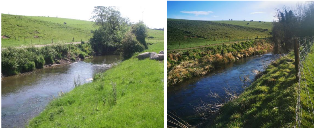
Figure 4.3 Photograph taken on the left-hand bank looking from T0 upstream to T30 (left, 2009 and right, 2022) where the vortex weir was constructed.
