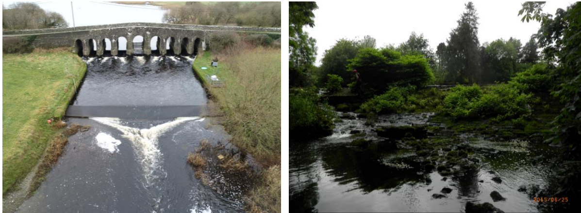
Figure 2.25 The nine-eye bridge at Stramatt with gauging weir downstream (left). Note Lough Ramor in the background. Virginia weir (right). Note the person in the left of frame for scale, demonstrating the extreme hydraulic head height.
