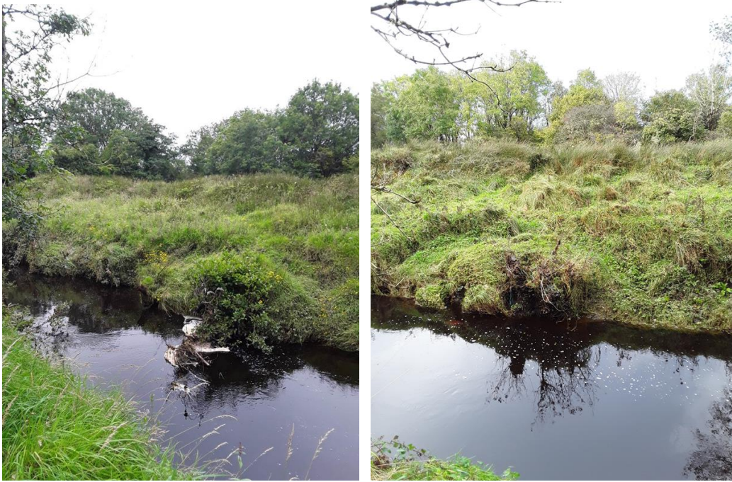
Figure 5.2 Example of an obstruction removed from the channel (left, 2020 & right, 2021).
