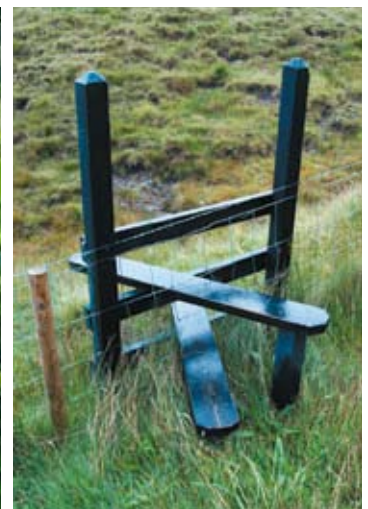
Stiles provide access over fences, but create difficulties for less mobile users. Killarney, Co. Mayo.
