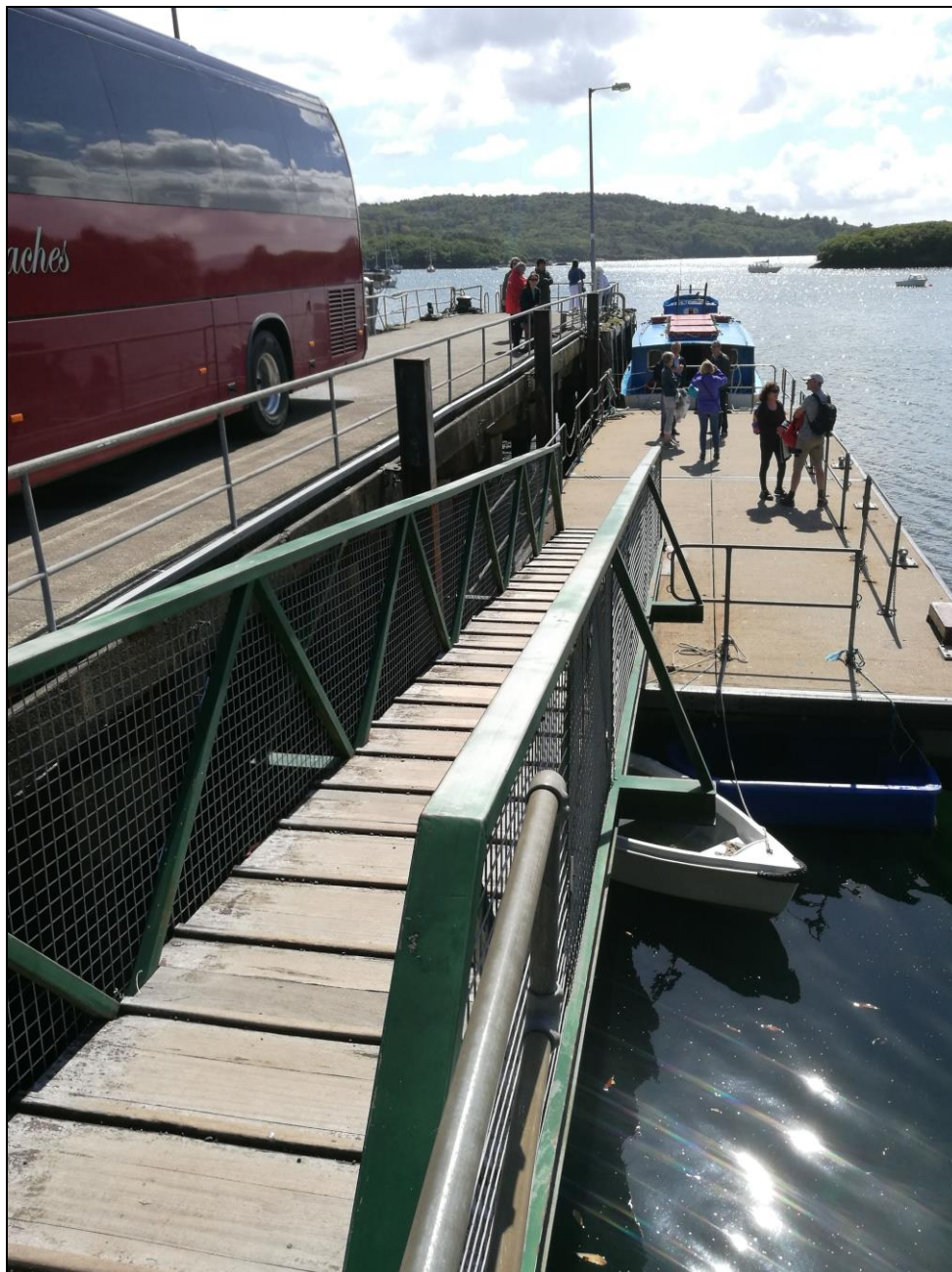
Plate 1. View of pontoon looking south-east from the gangway at Glengarriff Pier
