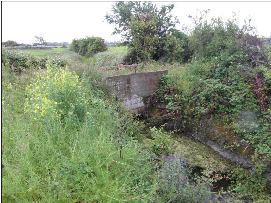
Photograph 4: View upstream looking downstream
