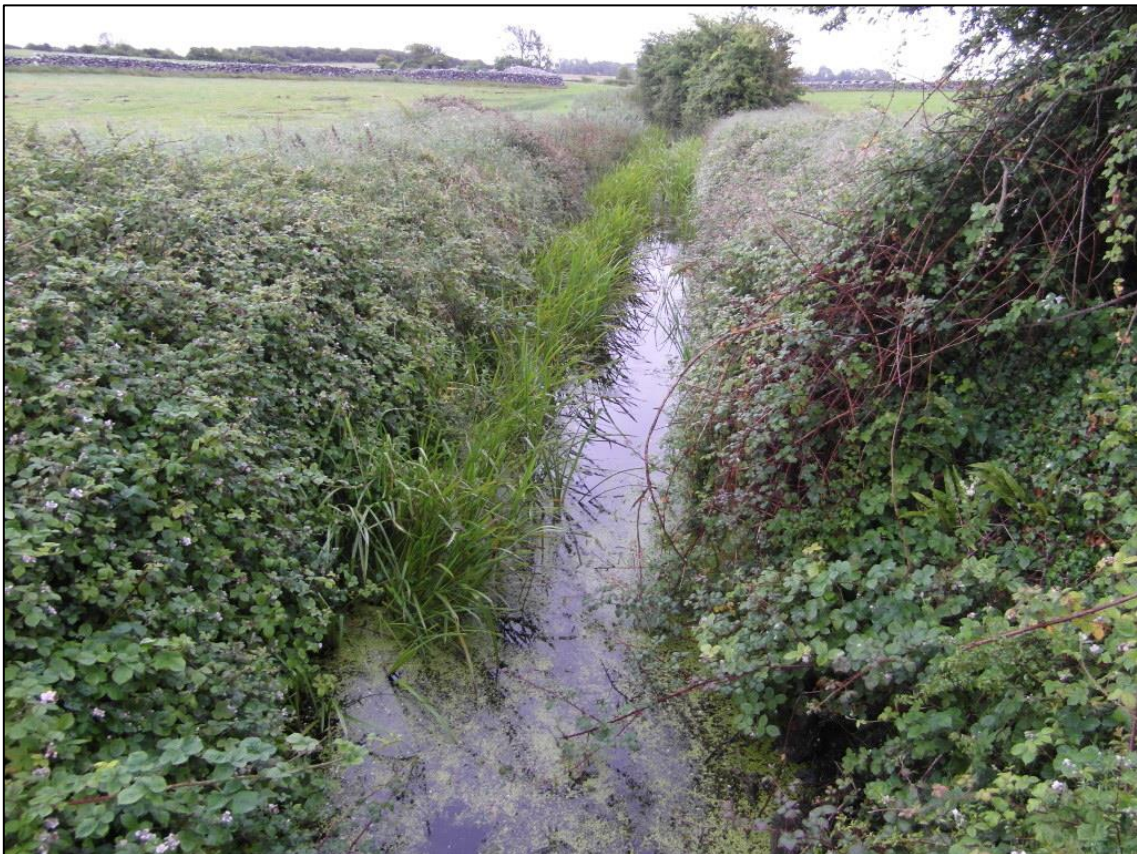
Photograph 2: View downstream of proposed new bridge
