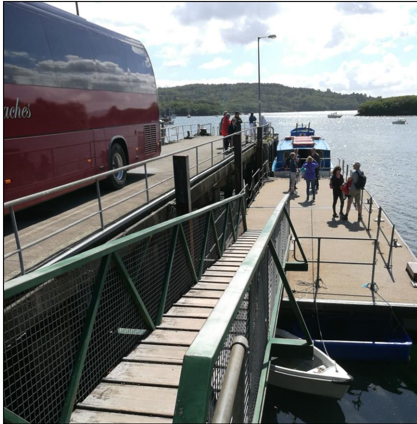
Plate 1. View of pontoon looking south-east from the gangway at Glengarriff Pier
