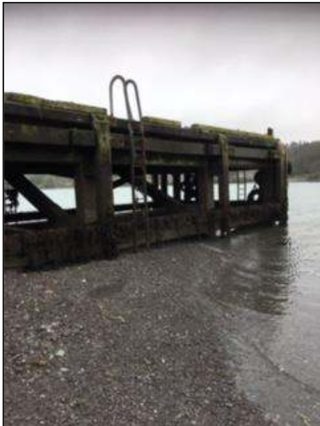
Plate 4: Reen Pier looking west
