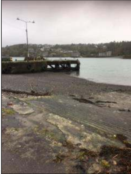
Plate 3: Reen pier looking west
