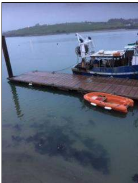
Plate 7: Courtmacsherry pontoon (to be temporary removed for dredging)
