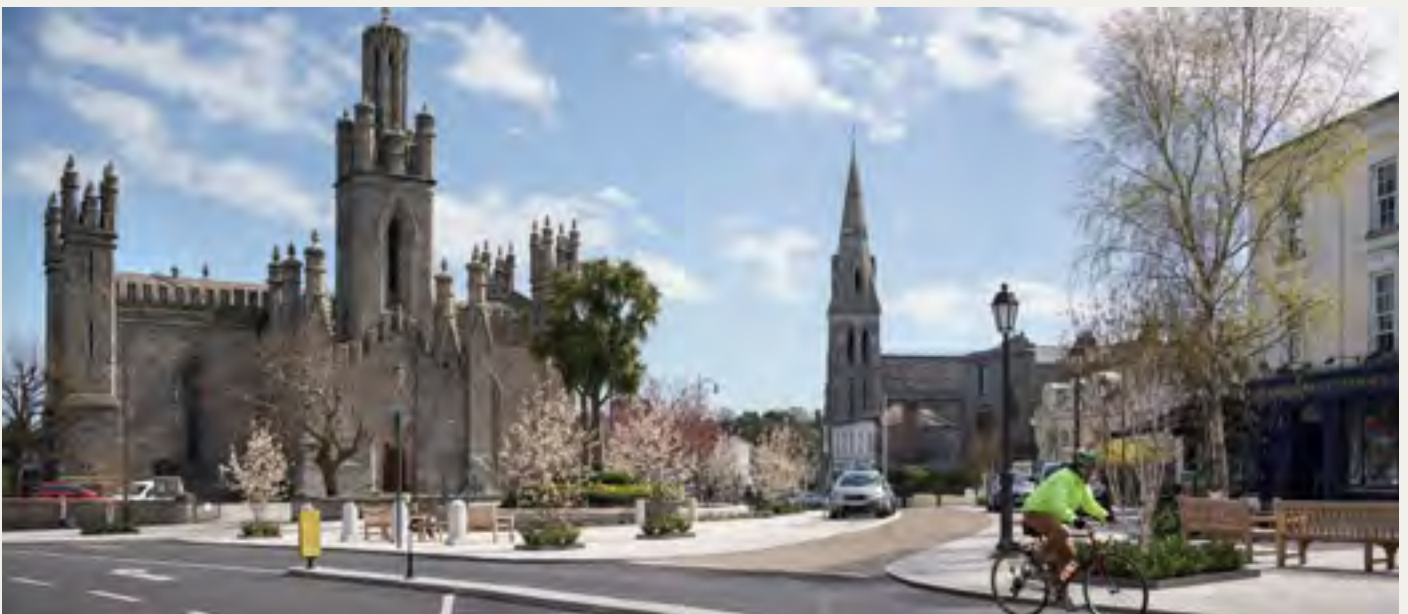
Tionscadal Shráidbhaile Bhaile na Manach, Contae Bhaile Átha Cliath. DLR Architects. Gearrliosta na nGradam RIAI, 2019. Grianghraf le Donal Murphy
