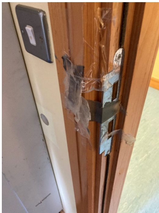
Figure 11: Computer Room, Pine Lodge
