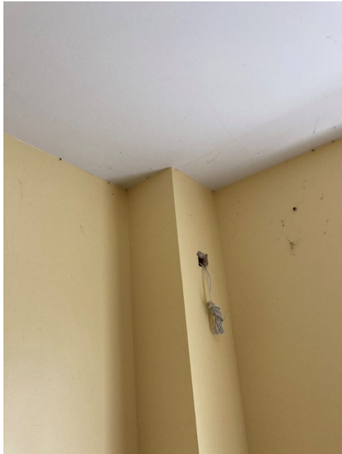
Figure 10: Computer Room, Pine Lodge
