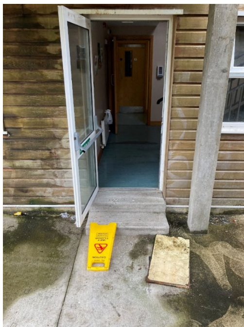
Figure 8: Fire Exit Doorway, Pine Lodge
