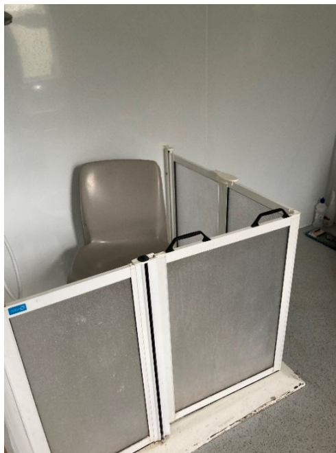
Figure 7: Wheelchair Accessible Shower Area, Pine Lodge
