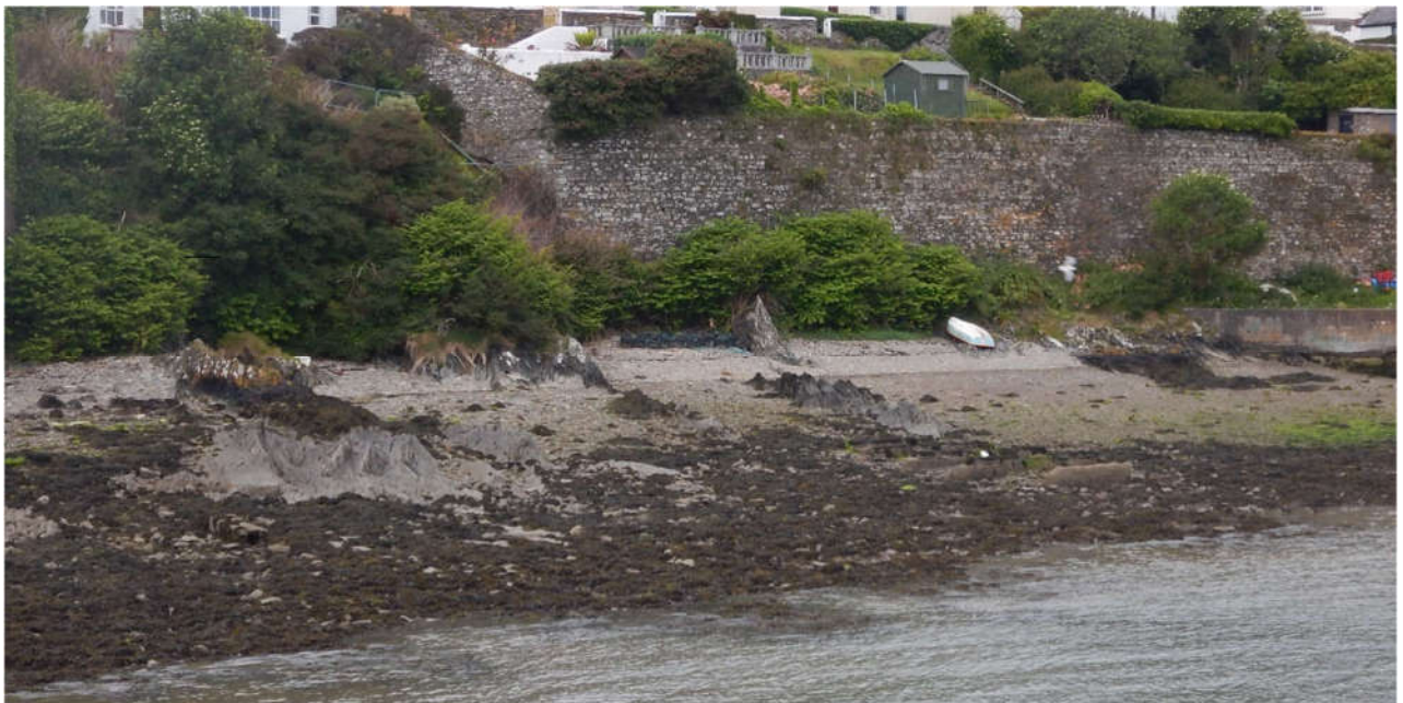
Figure 5.1 Stone walling along the south western boundary of Ballycotton Harbour.
