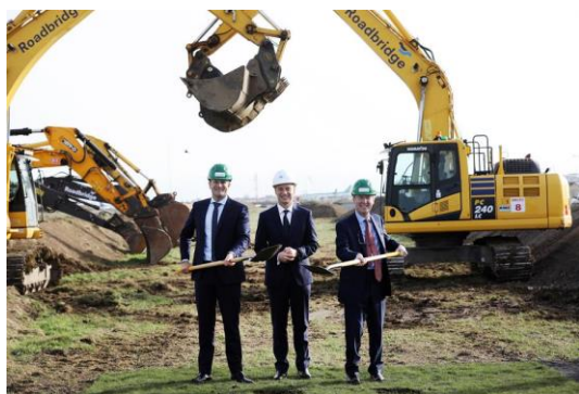
An Taoiseach, Leo Varadkar TD and the Minister for Transport Tourism and Sport, Shane Ross TD turning the sod for Dublin Airport's new North Runway project
