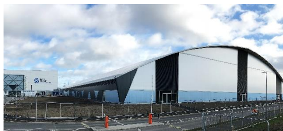
The National Indoor Arena is nearing completion.
